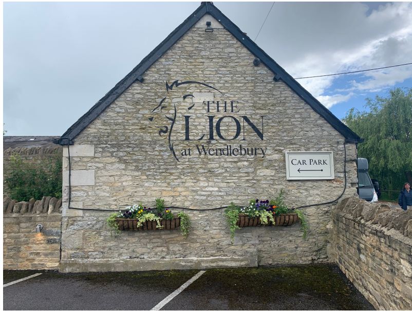
SIGNWRITING TO EAST GABLE - O/A DIMS - 220cm W X 150cm H ( 3.3m2 ) LARGEST LETTER HEIGHT - 46cm H 1no 50w LED floodlight
