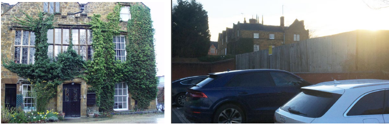
East Elevation/East and South elevations seen from car park.
