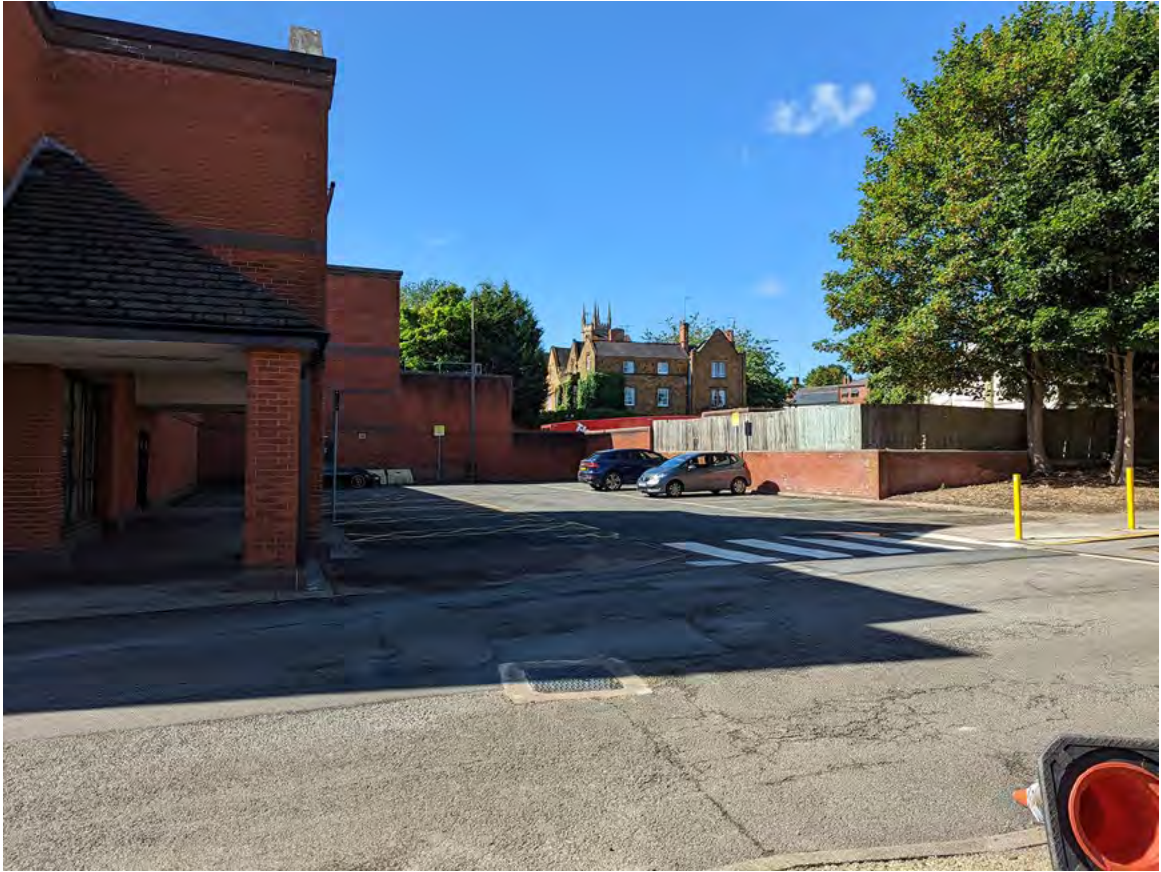
Plate 7: View of the western car park and Calthorpe House facing south-west
