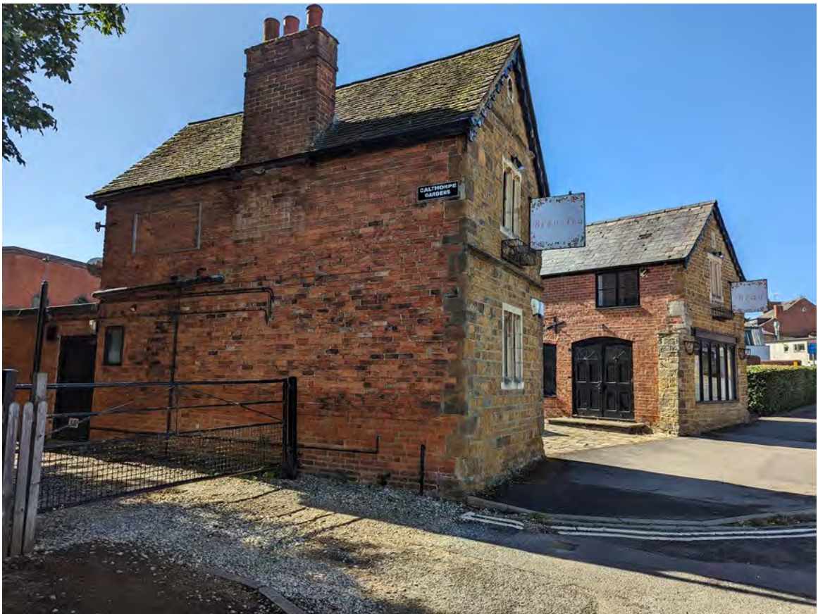
Plate 8: View of the Calthorpe gardens buildings facing south-east
