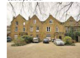
Gable end of Block AB
