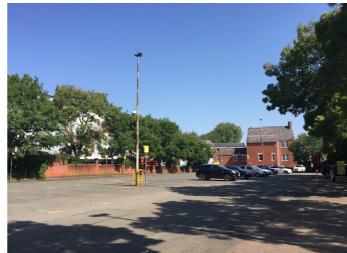
NCP Car Park and Retail Units
