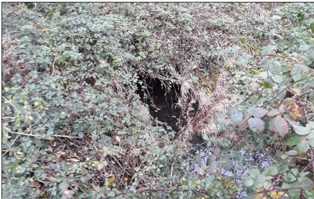
Figure 4.12: Photograph of Gallos Brook Channel at GB_00891
