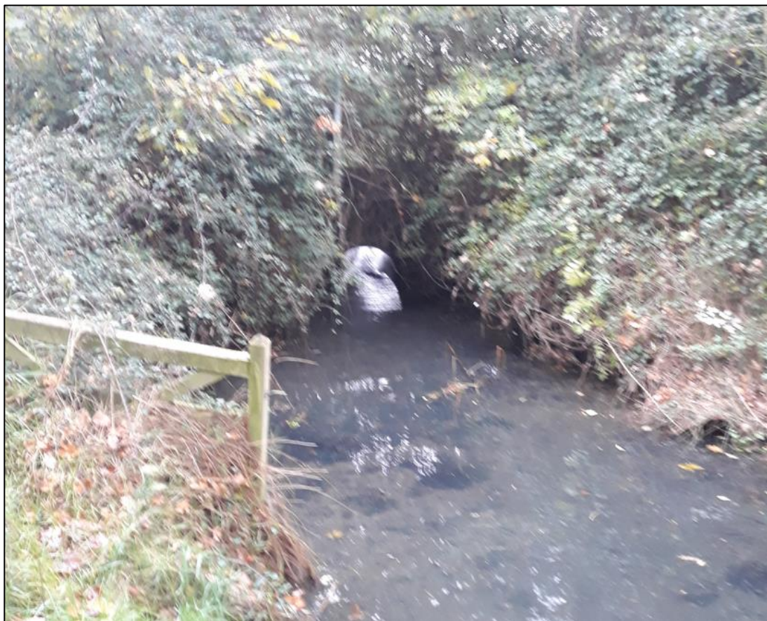
Figure 4.22: Photograph of Gallos Brook Channel at GB_01076
