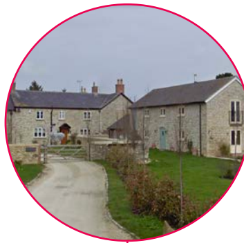
2 storey, barn style development, responding to the character of the development immediately to the west of the Site.
