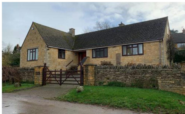
Bungalow at Junction of Woodway Road/Hook Norton Rd
