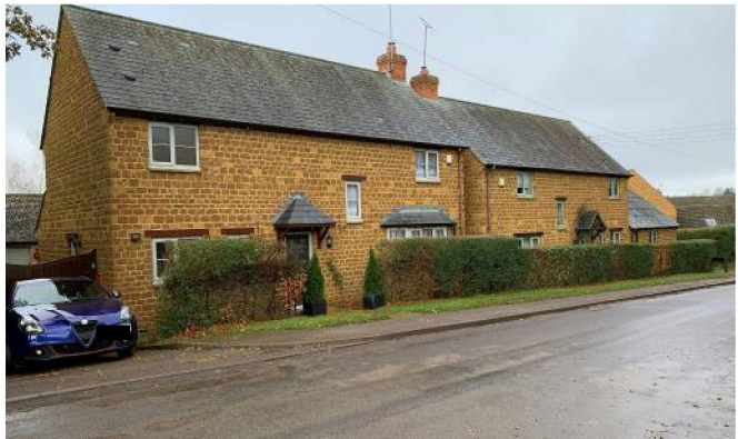
View west along Hook Norton Road/Stewarts Court
