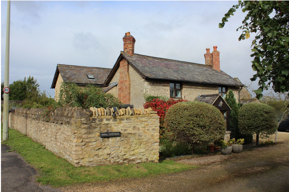
Image EDP 16: The south-facing historic façade and frontage of Pipal Cottage showing the brick angled chimneys and large rear northern 1980–1990s extension
