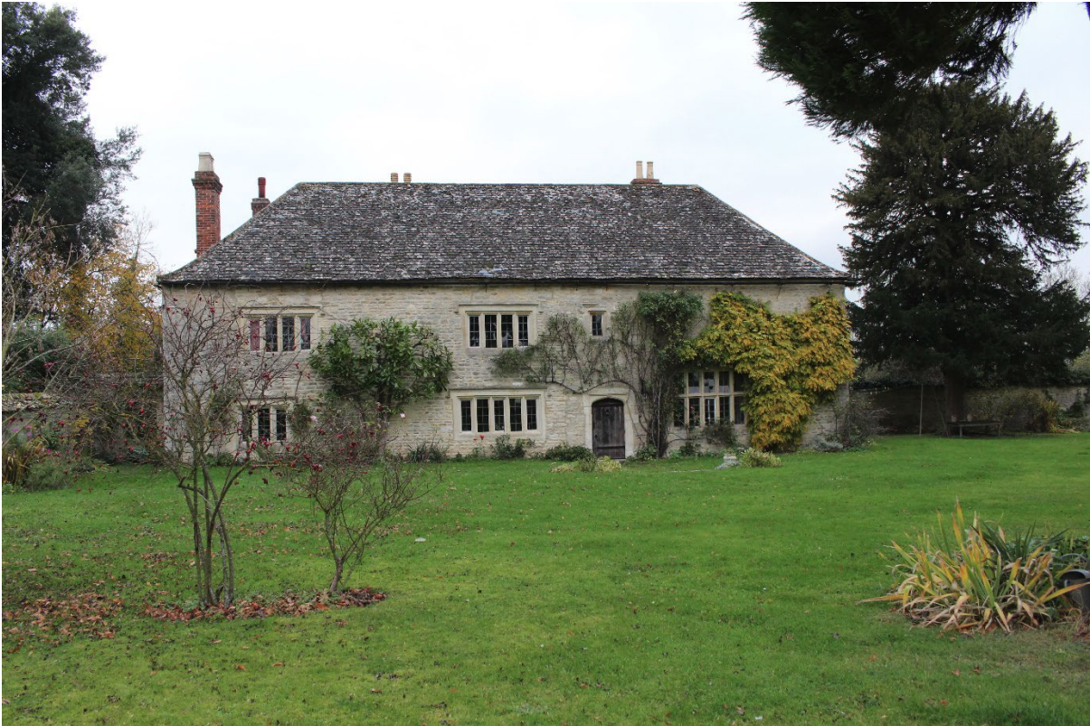
Image EDP 2: View of the principal southern façade of St Frideswide's Farm House, Grade II* listed building. The associated Grade II listed garden wall lies to the right of frame and this image illustrates the immediate and enclosed garden setting of the farmhouse.
