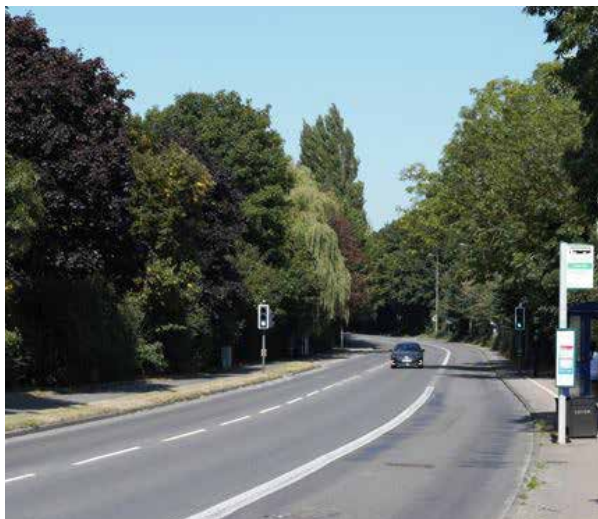
Extensive Boundary Vegetation to Oxford Road
