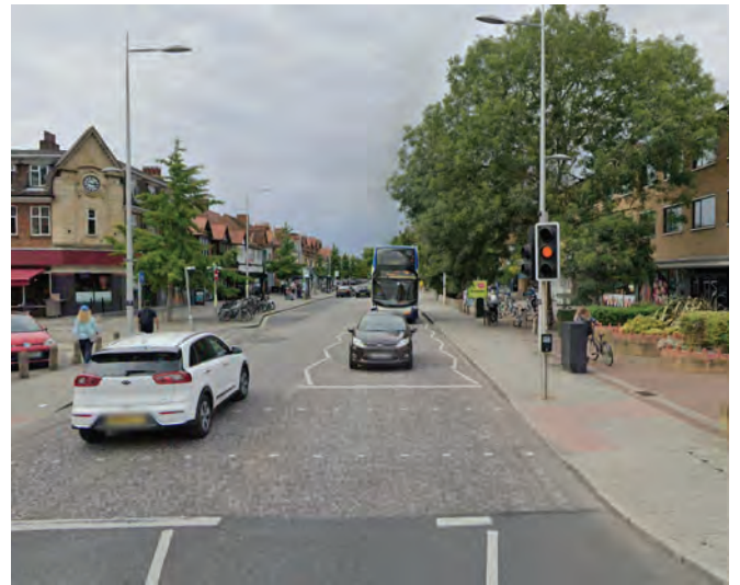
Oxford/ Banbury Road, Summertown
