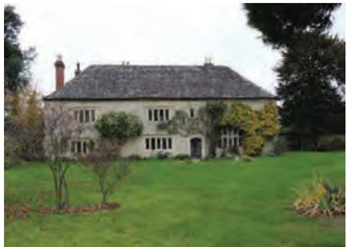
③ St. Frideswide's Farmhouse, Grade II* listed building
