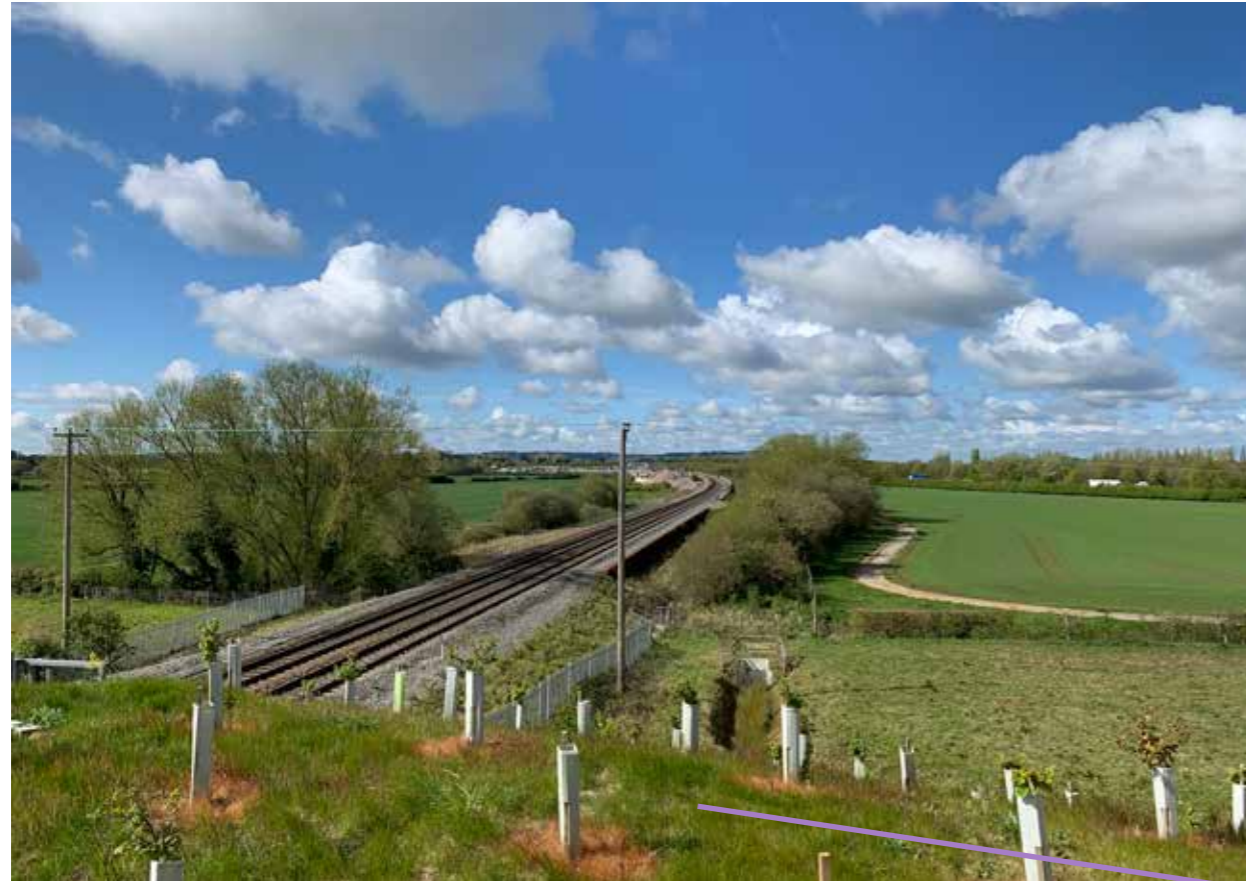
View from lane to Water Eaton, bridge over railway.
