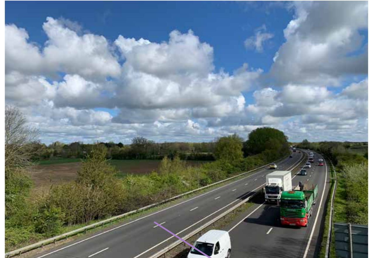
View from lane to Water Eaton, bridge over A34.
