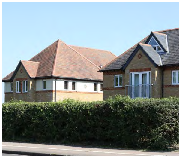
Development Context on Oxford Road
