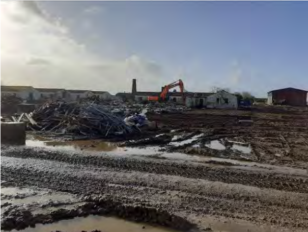
02.02.21 – Building demolition and hardstanding removal
