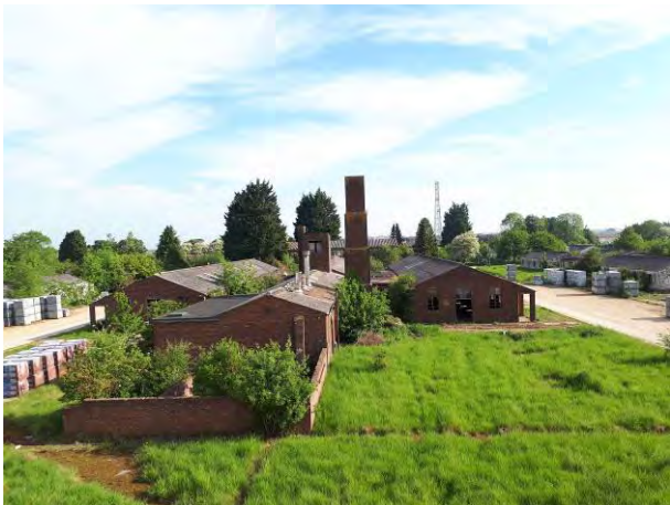
22.05.18 – Former boiler house in the centre of the site (chimney) with USTs
