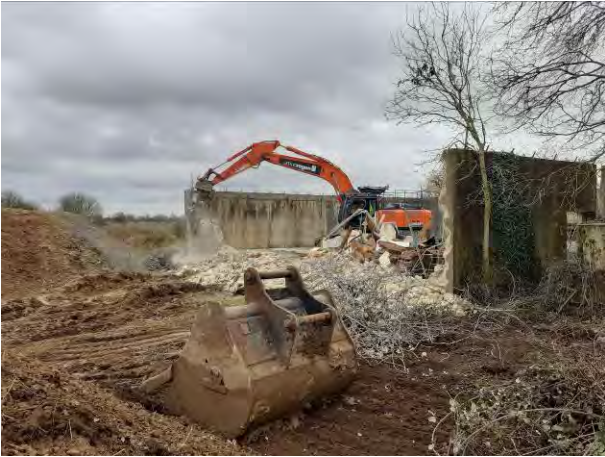
16.02.21 – Breaking out of walls around former substation
