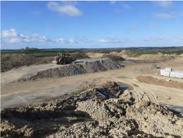
06.04.21 – Formation of site-generated aggregate stockpile (Agg-SP1) in the south
