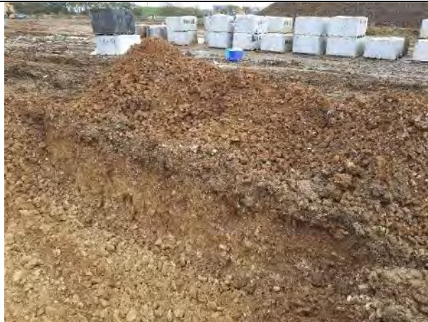
17.02.21 – Natural soils encountered from the surface to the base, consisting of limestone gravel in clay soil
