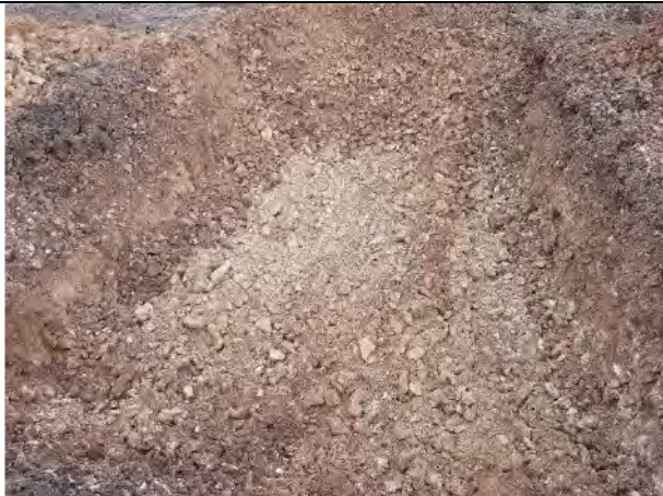
17.02.21 – Excavation of second trench to 1.1m bgl
