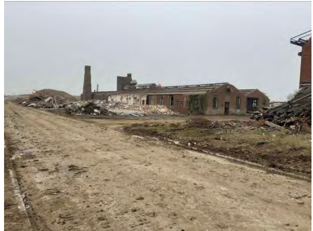
02.03.21 – ACM strip of boiler house complete, internal strip of boilers on-going
