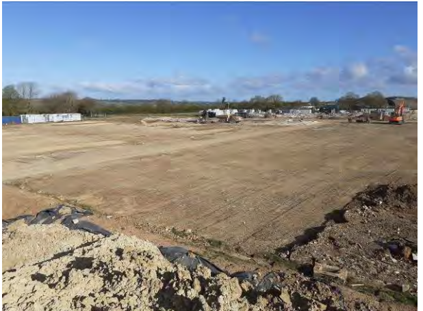
06.04.21 – North-western view across the site following building demolition and regrade
