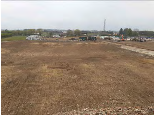
28.04.21 - Northern view across centre of site
