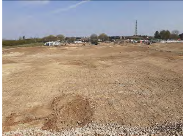
20.04.21 – Northern view across site
