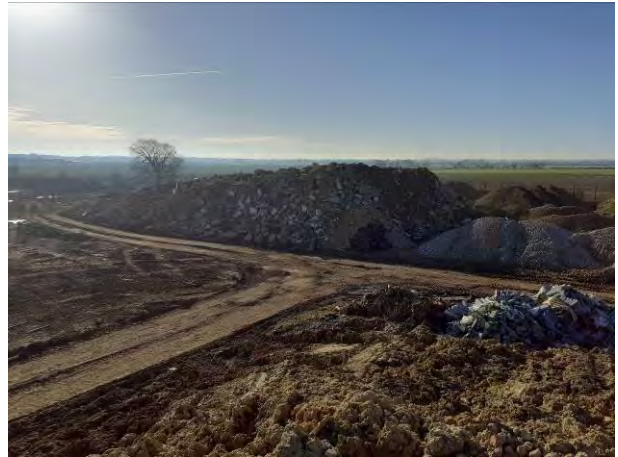
09.03.21 – Stockpile of recovered hardstanding awaiting processing to generate aggregate
