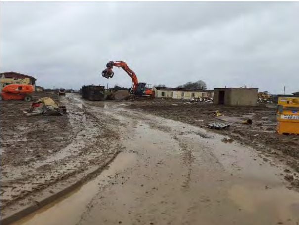
20.01.21 - Recovery and recycling of demolition materials
