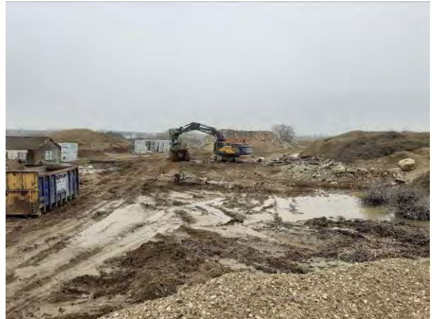
02.03.21 – Recovery of metal waste in to recycling skip in the southeast
