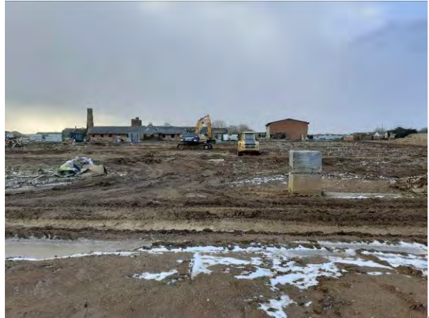
08.02.21 – Easternmost line of building demolished and hardstanding removal prior to surface level regrade
