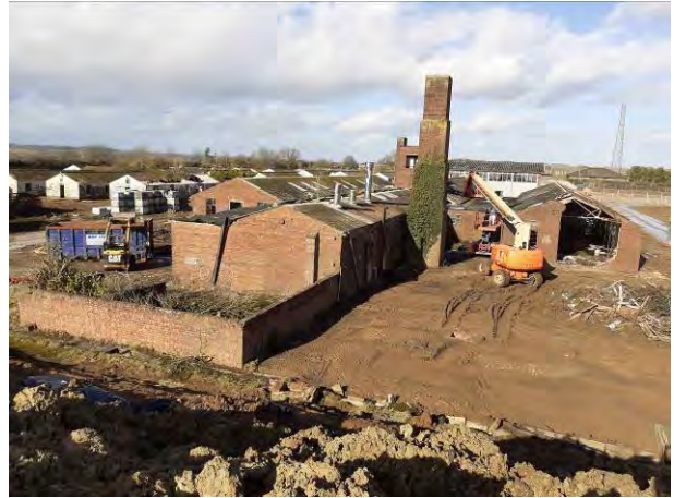
16.02.21 – ACM strip from boiler house
