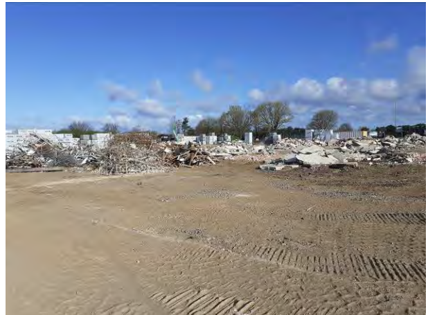
06.04.21 – Temporary stockpiles of wastes (metal, wood and masonry) prior to recovery
