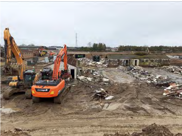
16.02.21 – Building demolition in south
