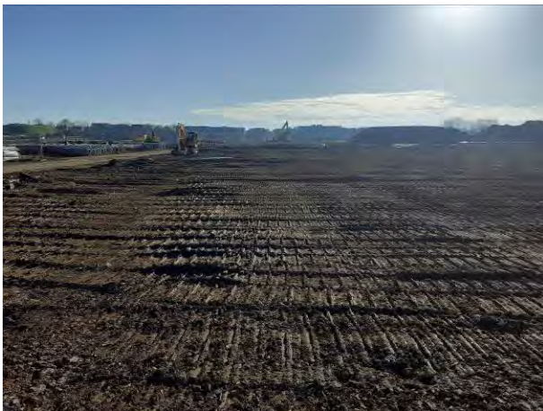
09.03.21 – Eastern view following regrade completion
