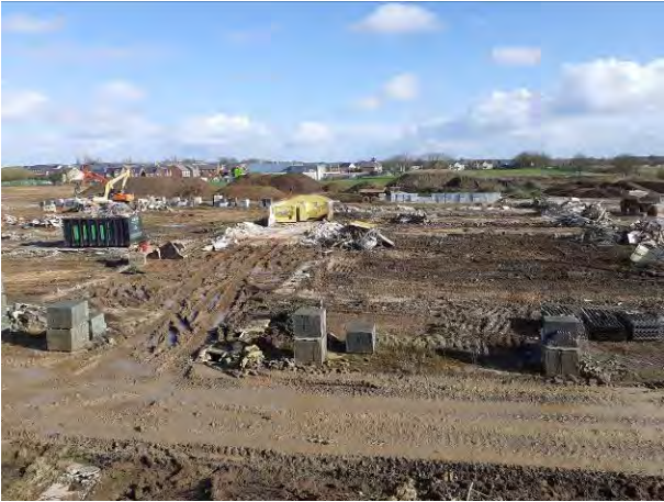
16.02.21 – Eastern view across site within area of recent building demolition
