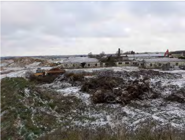
08.02.21 – Western view across site from eastern boundary
