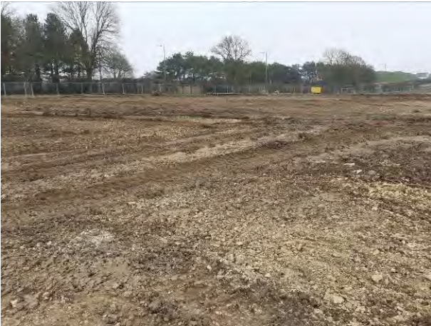
02.03.21 – Formation soils ready for sampling in northeast of site
