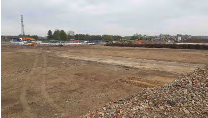
13.05.21 – North-eastern view following completion of works
