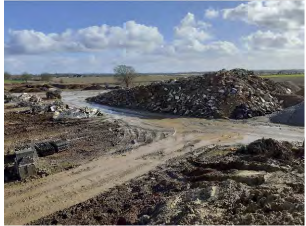
16.02.21 – Stockpile of recovered hardstanding prior to processing
