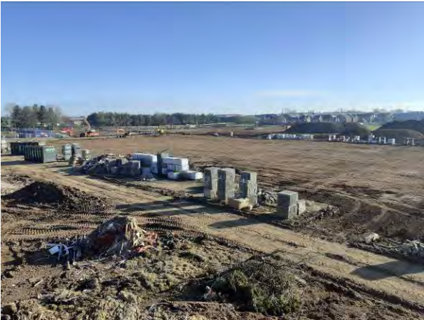
09.03.21 – Eastern part of the site trimmed awaiting formation testing
