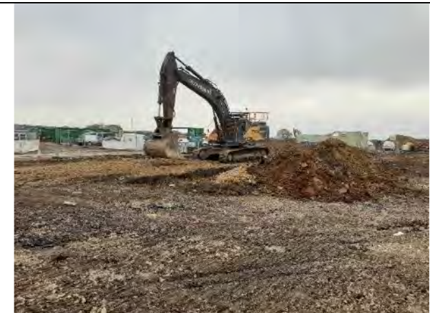
28.04.21 – URL removal of black stained gravel
