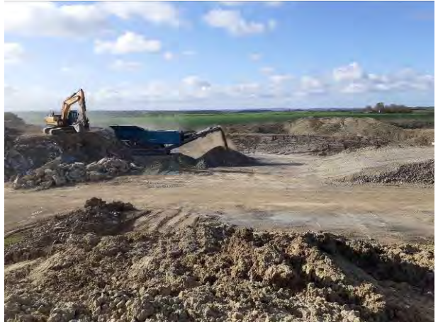
06.04.21 – Crushing site-won hardstanding commencing
