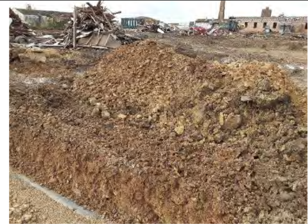
17.02.21 – Arisings side cast and consisted of coarse limestone gravel in brown clay (weathered bedrock). No visual or olfactory evidence of contamination, PID <0.1ppm.
