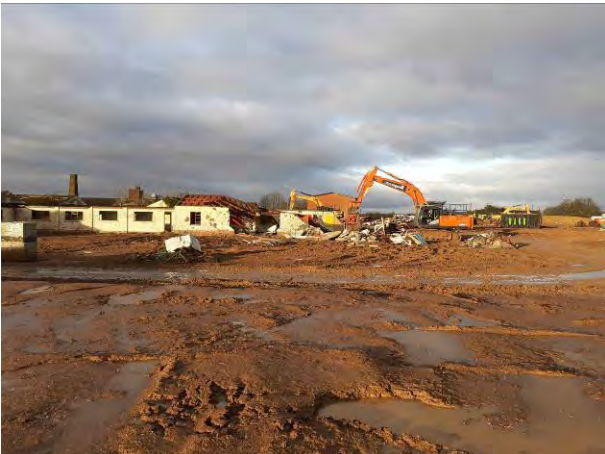
02.02.21 – Building demolition in north
