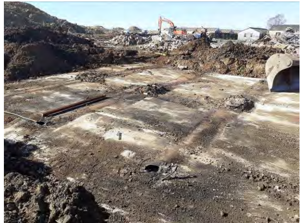
09.03.21 – Exposure of USTs following demolition of boiler house
