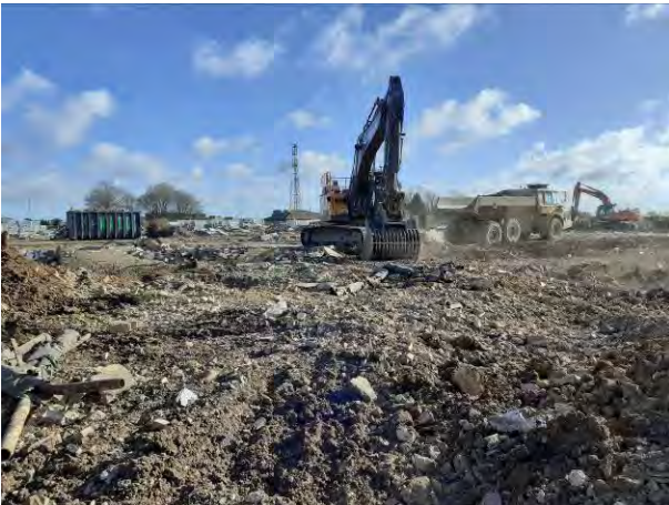
06.04.21 – Recovery of demolition waste materials in the north
