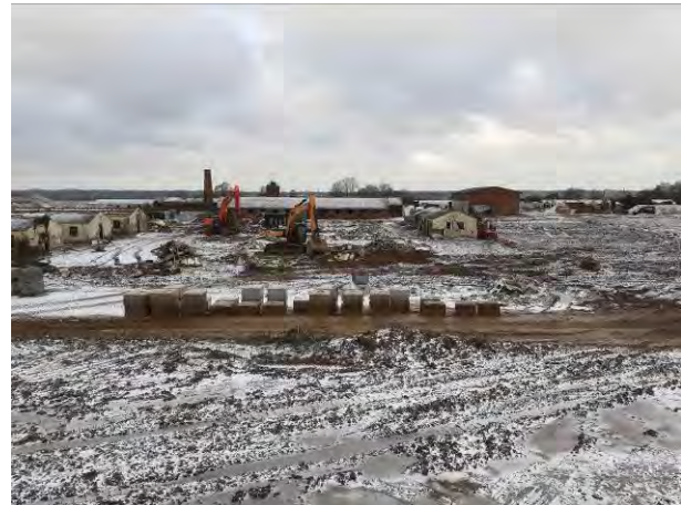
08.02.21 – Regrading to east of boiler house
