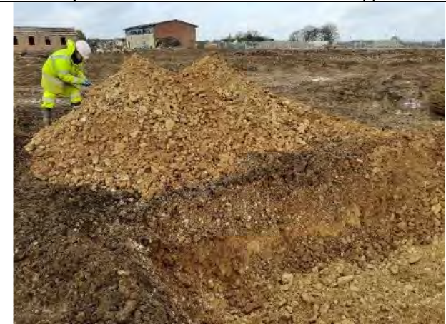
17.02.21 – Inspection of arisings and collection of validation samples. No visual or olfactory evidence of contamination, PID <0.1ppm.
