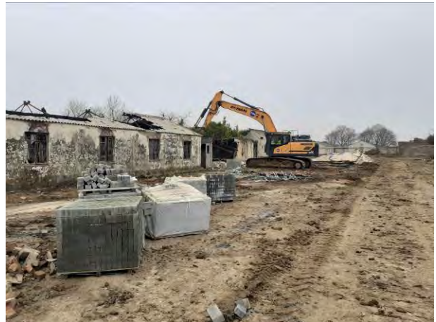
02.03.21 – Demolition of buildings in north/centre of site following ACM strip
