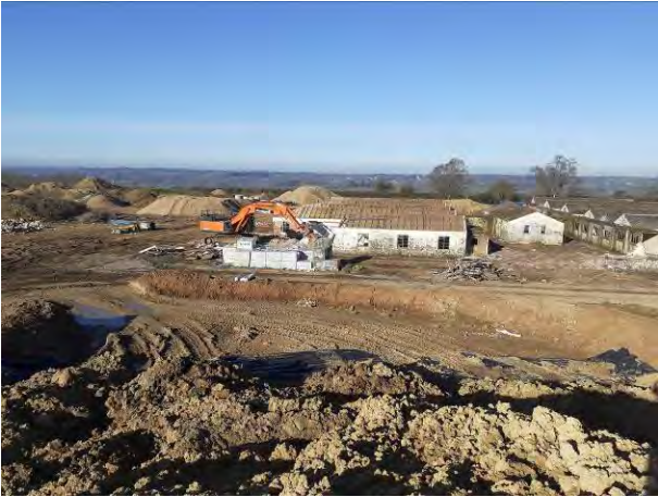
09.03.21 – Western view across the southern half of the site
