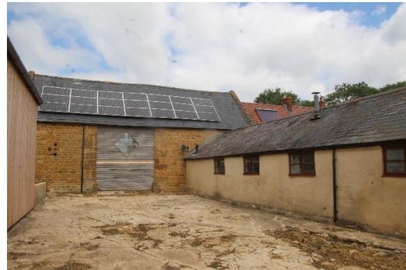
16. Barn and enclosed yard from the south
