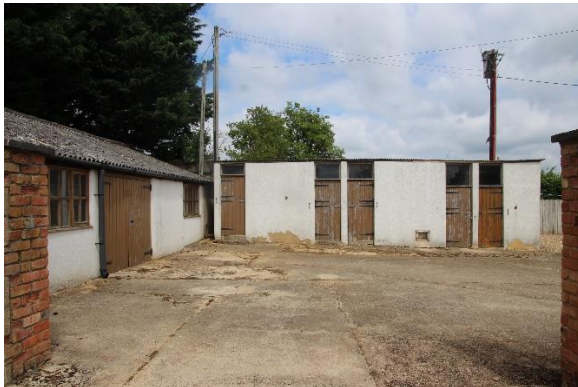
15. Stables in north-west corner of site
