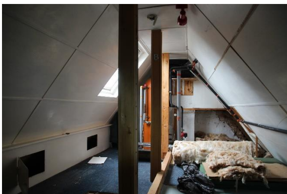
7. Western vaulted roof space of main house
