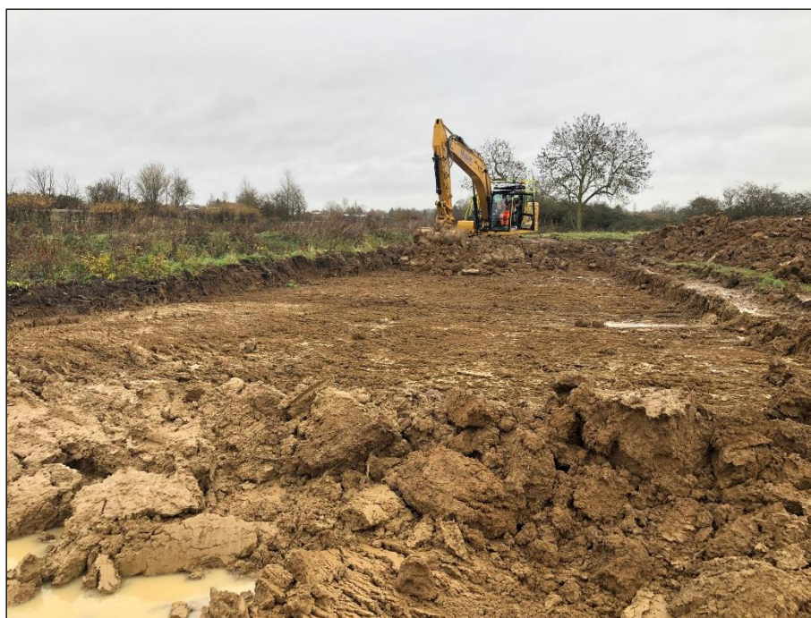
Plate 4: Post-excitation view after topsoil strip at north east corner, looking northeast
