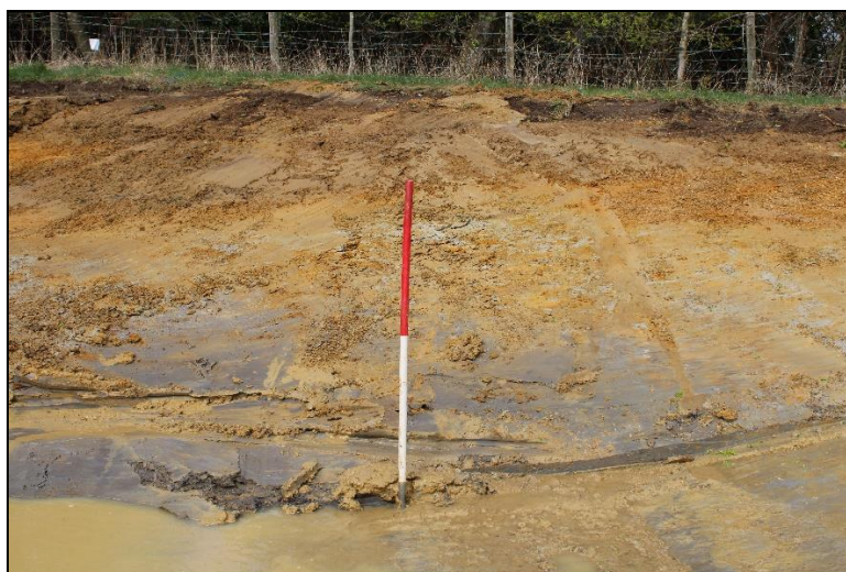
Plate 9: Representative Section of River Diversion, looking west.
