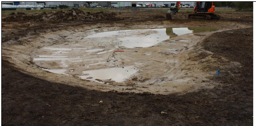
Plate 3: General view of Pond 2, looking south.
