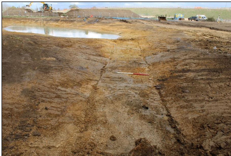
Plate 8: General view of River Diversion, looking north.
