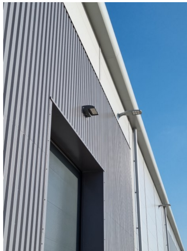
Vertical metal profile cladding & loading door
