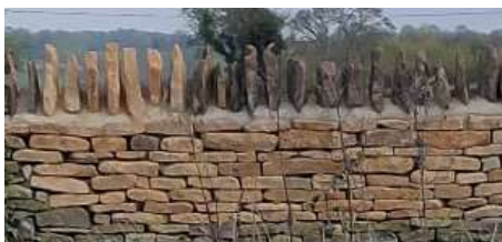
Fig.4: Looking due South, a short section of the limestone wall, referred to as a brick wall in the application. It is also not a very high wall.
