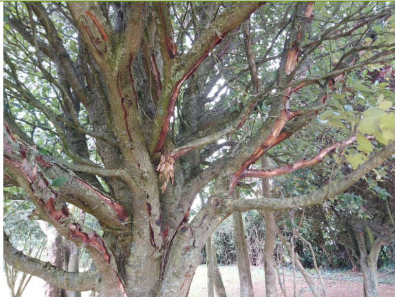
P1. Extensive fire damage to the structural framework of the whitebeam within G1.
