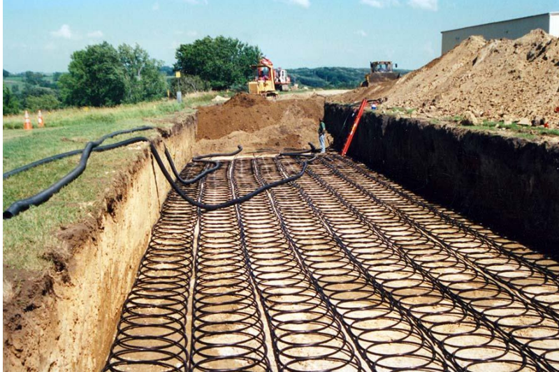
Figure B.4: Ground source heating horizontal collector loops being installed
