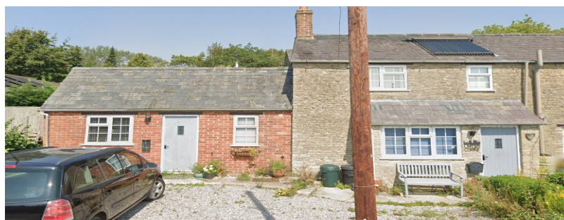
Figures 5, 6 and 7 – Properties along Wendlebury Road and Oxford Road, Wendlebury
