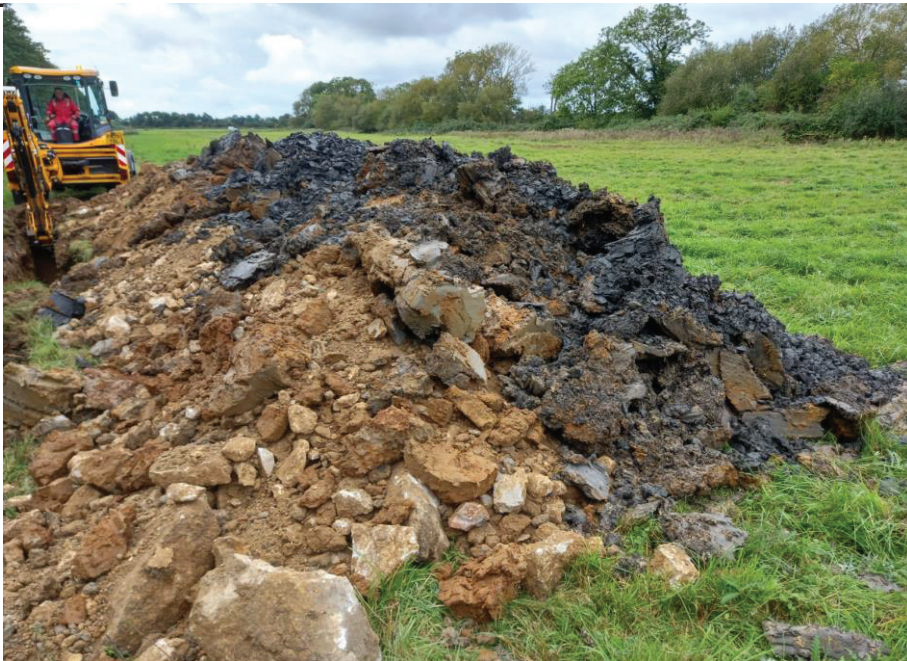
Trial Trench 1 Spoil
