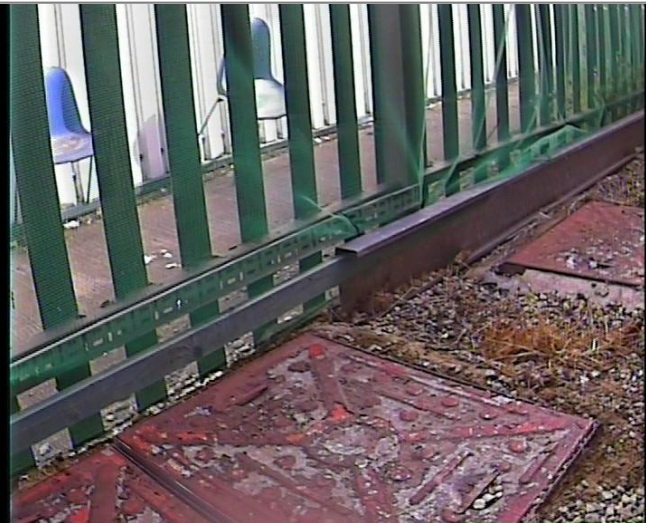
Manhole / Access Point: F4 Location
