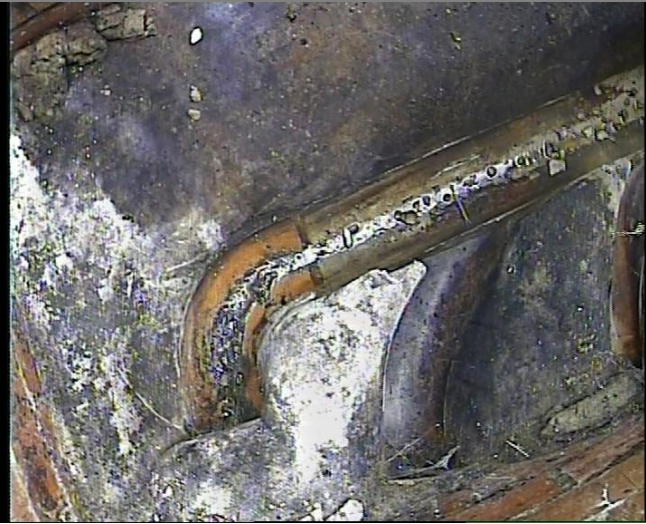
Manhole / Access Point: F3 Internal
