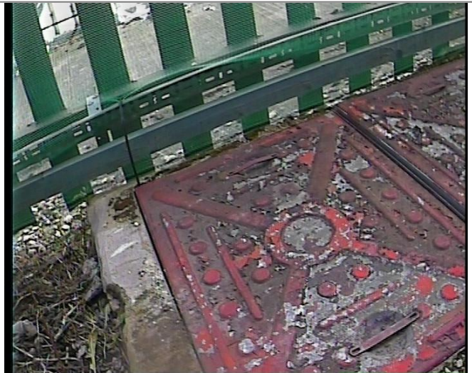
Manhole / Access Point: F3 Location
