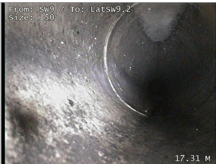
Settled deposits fine 5% cross-sectional area loss, Finished
