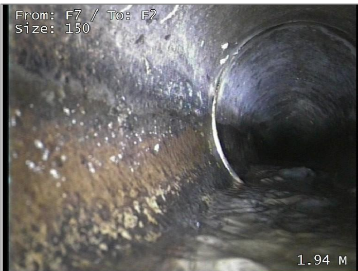
Other attached deposits from 7 to 5 o'clock 5% cross-sectional area loss - Remark Scale, Start
