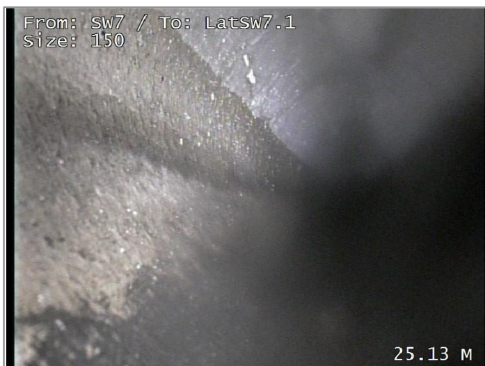
Survey abandoned - Remark: Unable To Push Further
