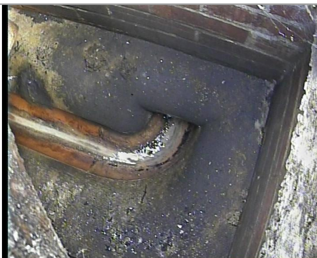
Manhole / Access Point: F1 Internal
