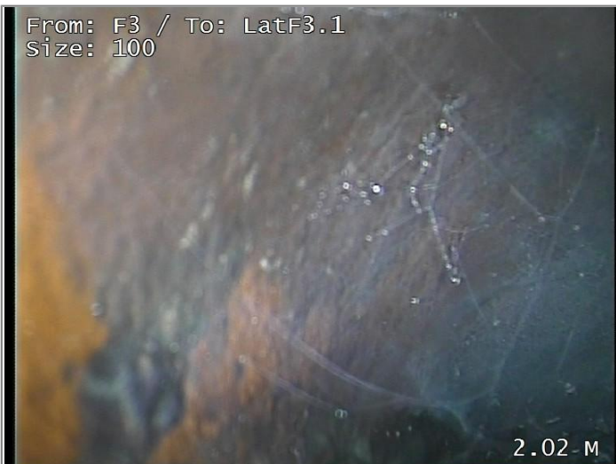
Settled deposits fine 5% cross-sectional area loss, Finished
