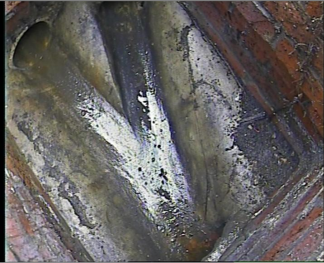
Manhole / Access Point: SW1 Internal
