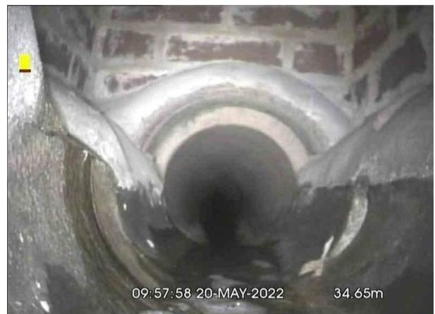
SW7X_8d4e9691-90da-42e4-aa06-2722d46ca9f2_20220524_155733_967.jpg, 00:01:35, 34.65 m Finish node type, manhole, reference number: SW7a, internal
