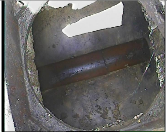
Manhole / Access Point: SW4 Internal
