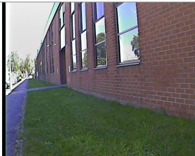
Access problems: SW4 - Far left of building
