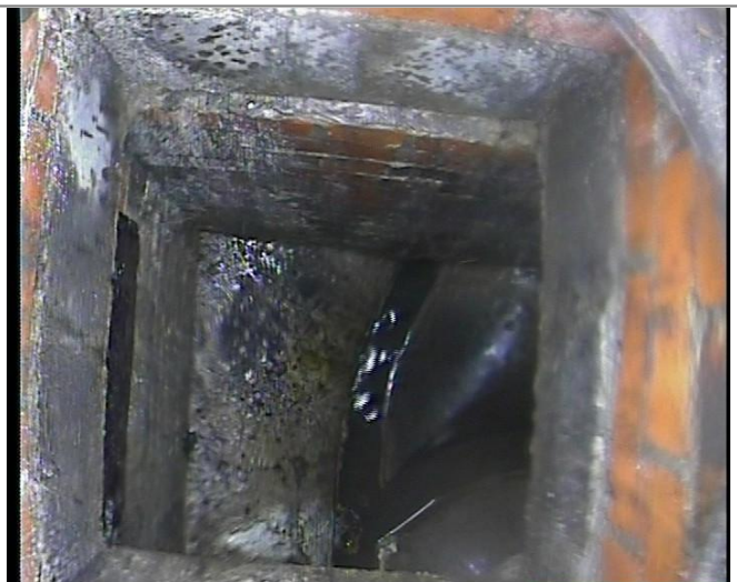
Manhole / Access Point: F5 Internal
