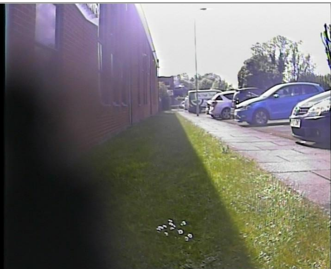
Manhole / Access Point: SW7 Location
