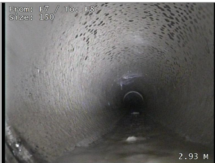
High rate of flow from upstream
