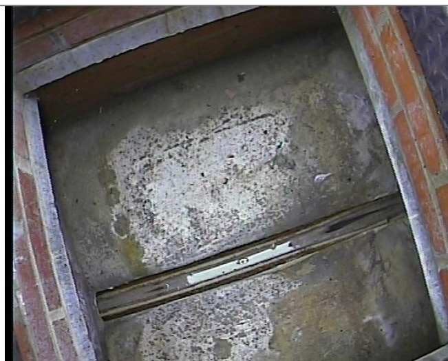
Manhole / Access Point: F6 Internal
