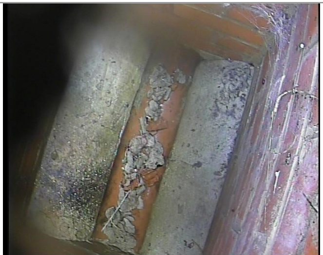
Manhole / Access Point: SW8 Internal
