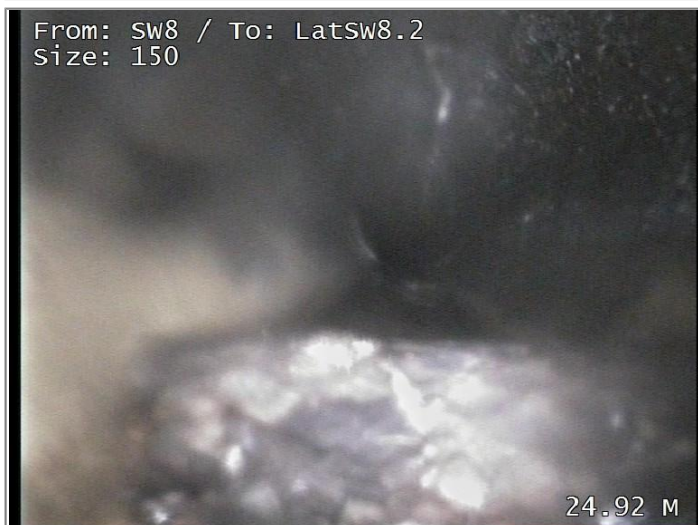
Survey abandoned - Remark: Unable to push further
