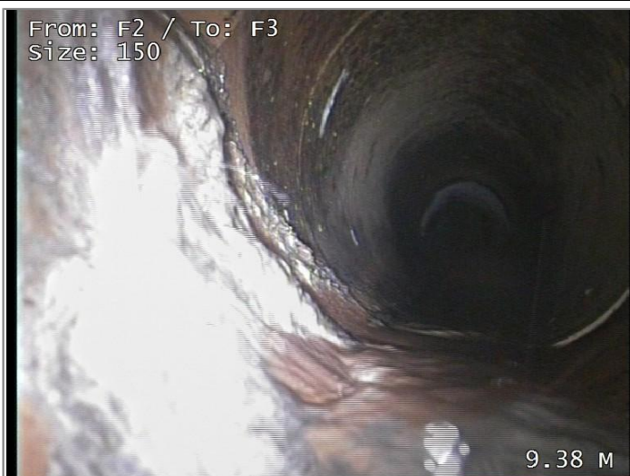
Other attached deposits at 10 o'clock 5% cross-sectional area loss - Remark Scale
