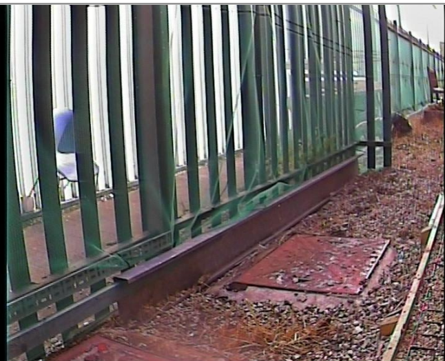
Manhole / Access Point: F5 Location
