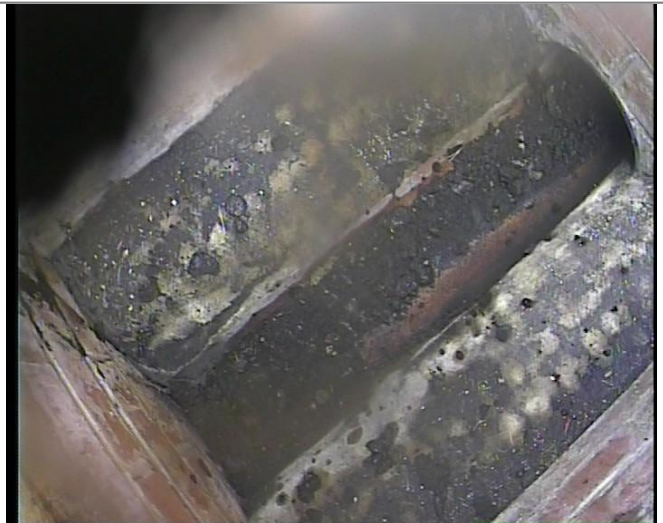
Manhole / Access Point: SW7 Internal
