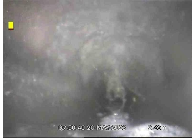
SW8aX_af97abca-b69c-4581-80f3-69327043c02c_20220524_155111_170.jpg, 00:00:19, 2.26 m Water level, 10% of the vertical dimension, froth on water?
