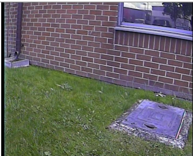
Manhole / Access Point: SW9 Location
