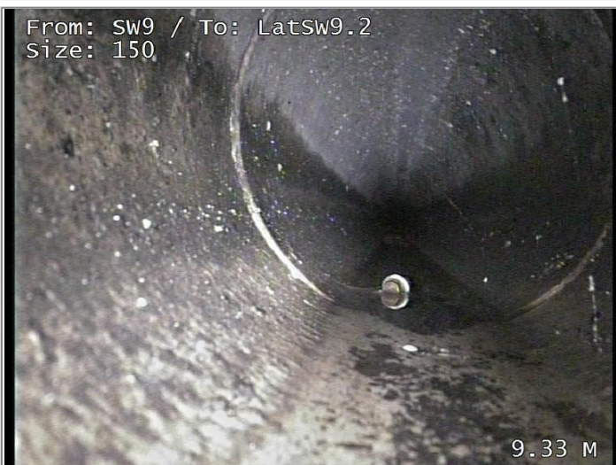
Settled deposits fine 10% cross-sectional area loss, Finished
