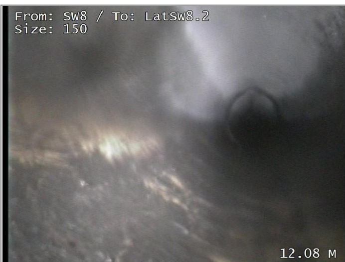
Settled deposits fine 5% cross-sectional area loss, Finished
