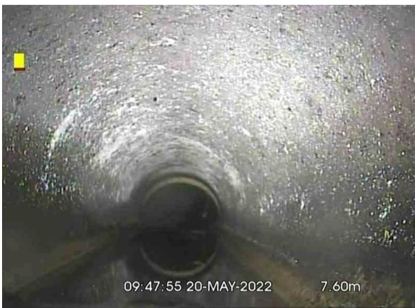
SW8X_342466c4-9ade-445f-b00d-9a2e7e0cc48a_20220524_154336_648.jpg, 00:00:33, 7.60 m Water level, 15% of the vertical dimension
