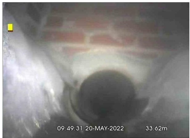
SW8X_21172983-4912-4885-a99f-58da5612fb49_20220524_154854_773.jpg, 00:02:09, 33.62 m Finish node type, manhole, reference number: SW8a, internal
