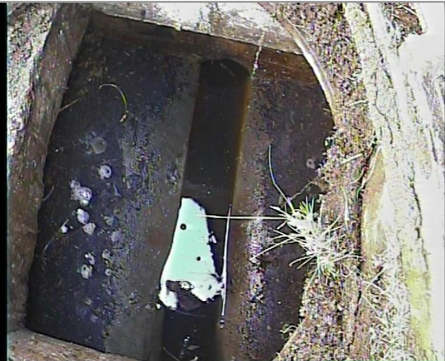
Manhole / Access Point: SW5 Internal
