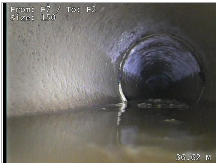
High flow rate through pipework
