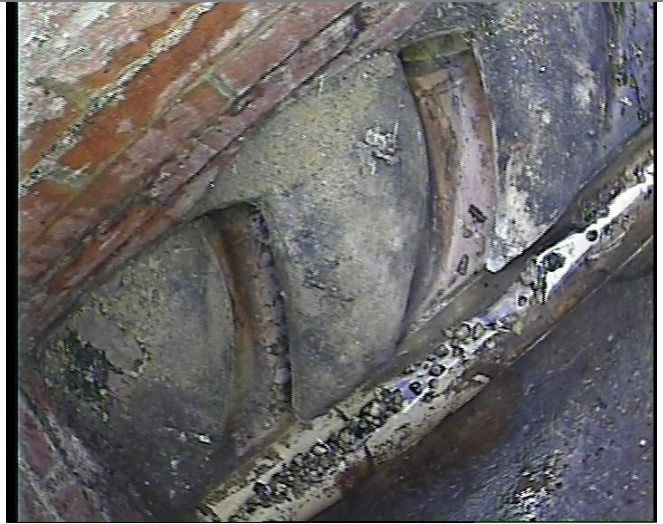
Manhole / Access Point: F4 Internal
