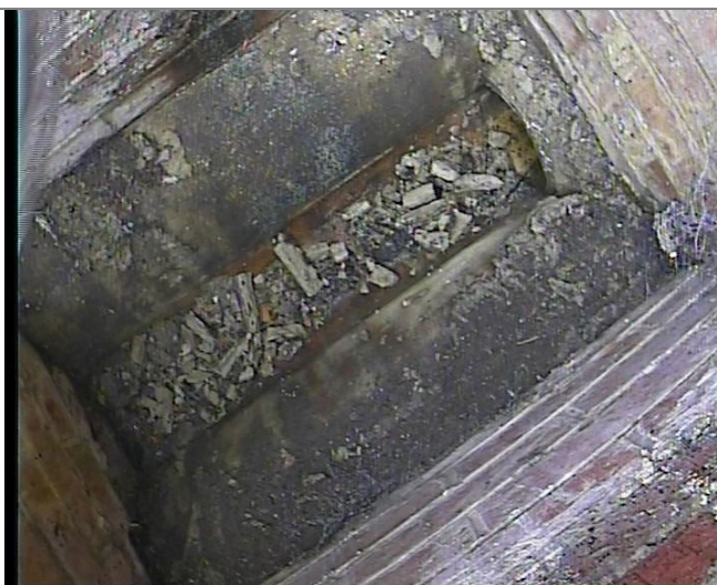
Manhole / Access Point: SW9 Internal
