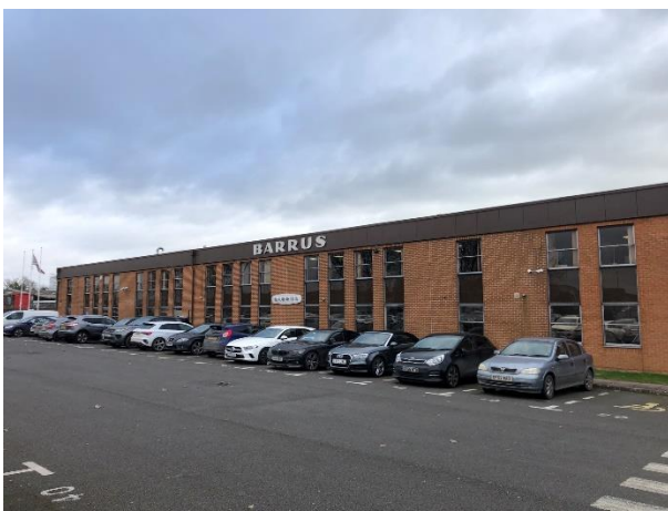
Fig 02 – Photo of existing building.
