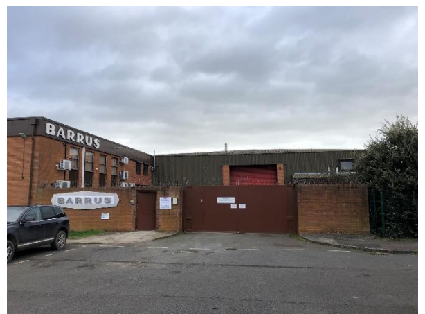
Fig 05 – Existing Service Yard.
