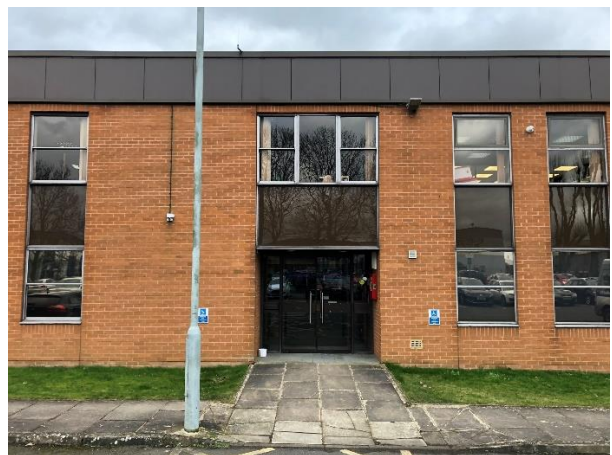
Fig 07 – Existing building entrance.
