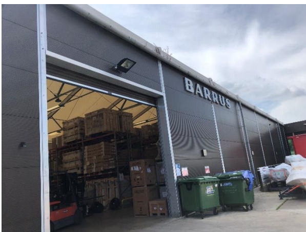
Fig 04 – Existing Rubb Type Building.
