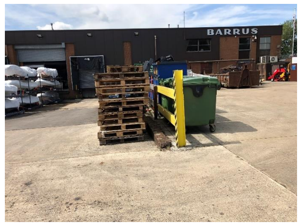
Fig 03 – Existing Delivery Yard.
