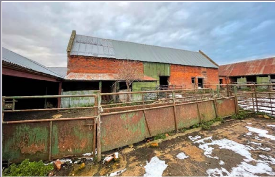
NORTH RANGE, SOUTH ELEVATION
