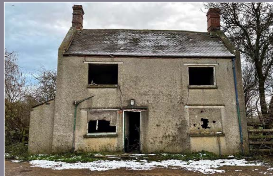
HUSCOTE FARMHOUSE, NORTH ELEVATION
