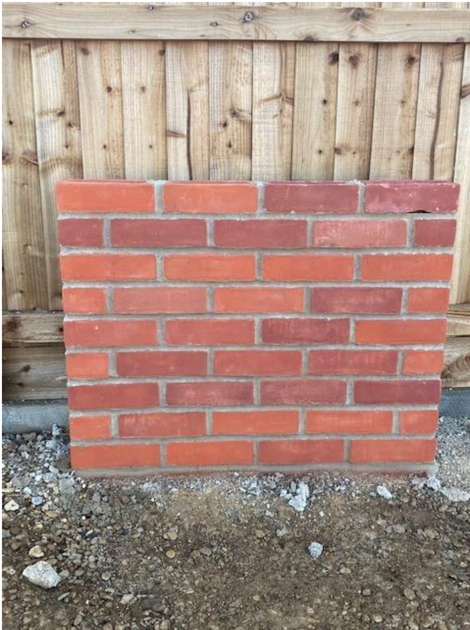
Brick Sample Panel
