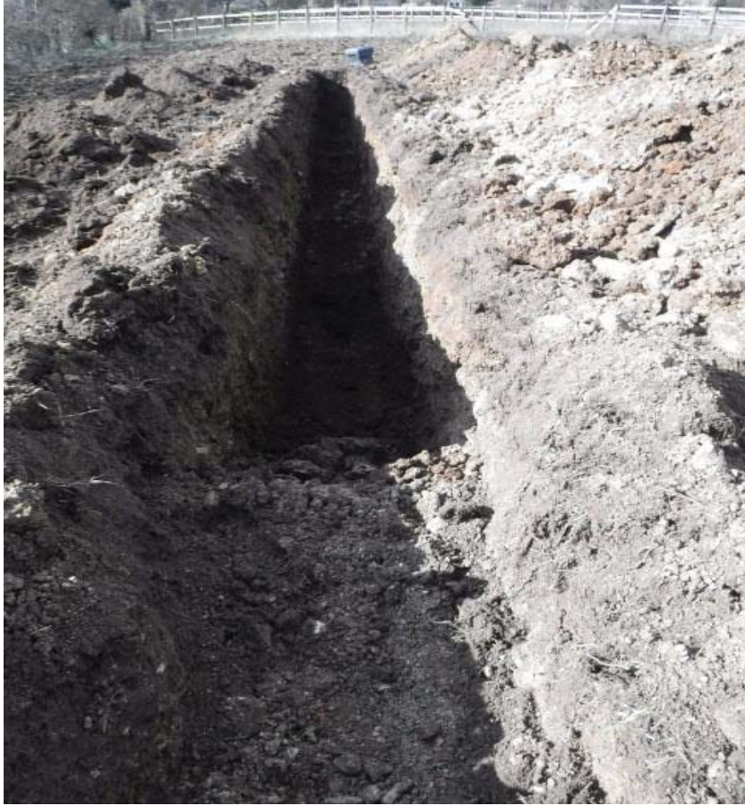
Trial Trench TP15 looking North West
