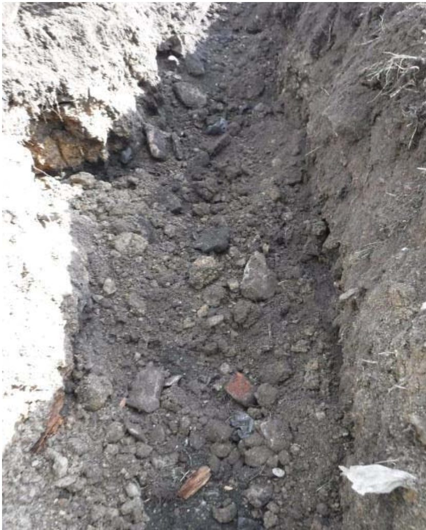
Trial Trench TP16
