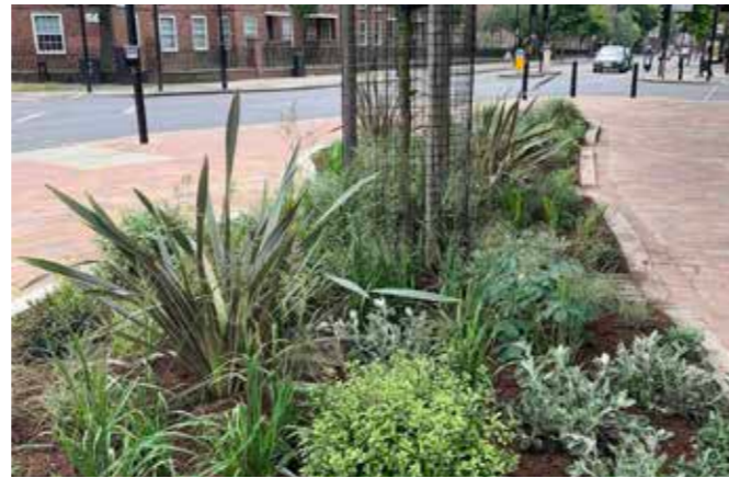
Raingardens within shared surface Lanes
