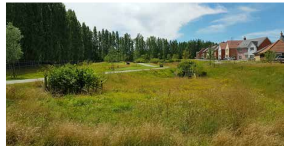
Attenuation basin on the edge of housing
