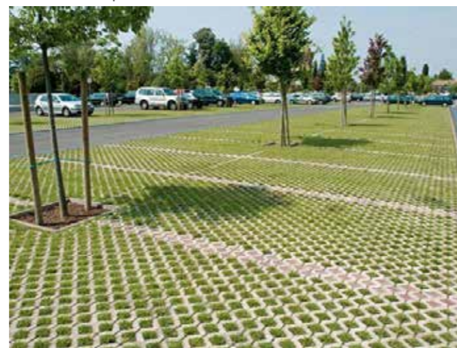
Reinforced grass parking area
