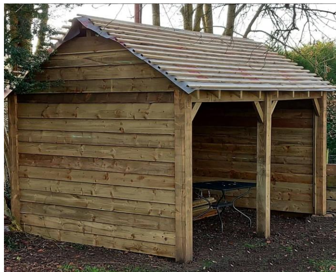
Fig. 1 Open-fronted garden store
