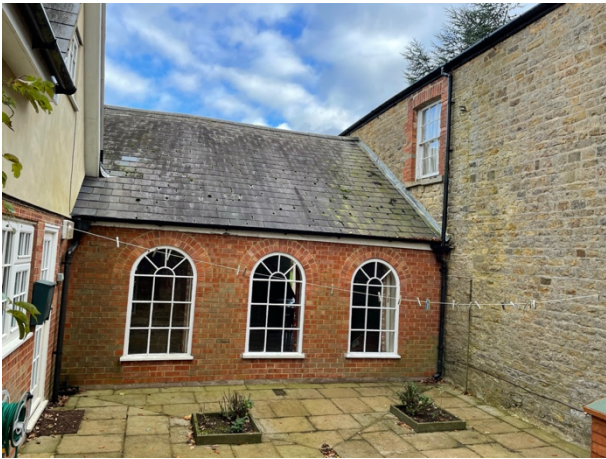
Wall and roof to be removed.
