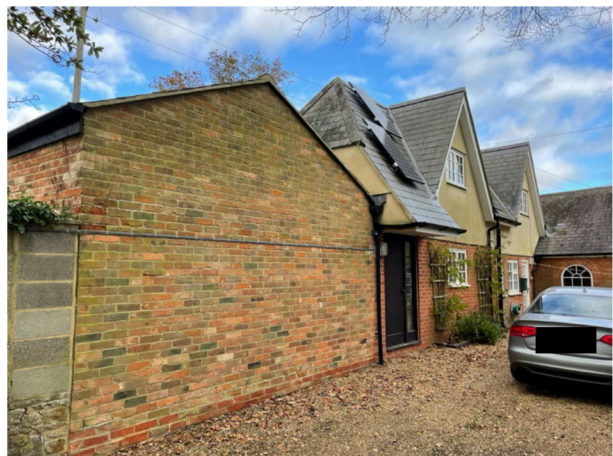
South facing 2 storey extension.
