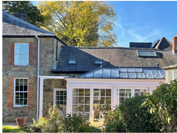
Wall to be raised, window added, new roof over.
