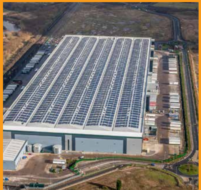
Photo courtesy Amber infrastructure
