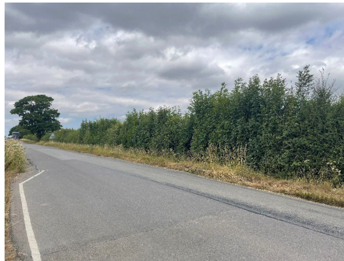
Plate 4: Tall hedgerow at the southern boundary of the site, looking north-west from same location as Plate 3
