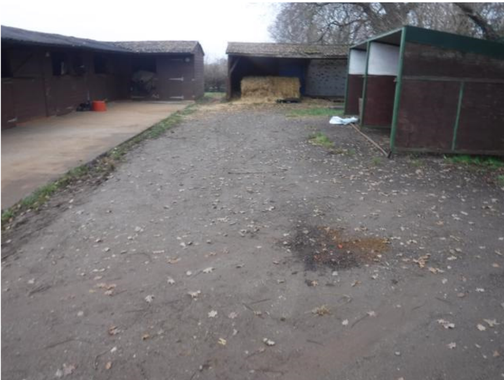
Stable Block looking Northerly. Backfilled HP3 in the foreground.
