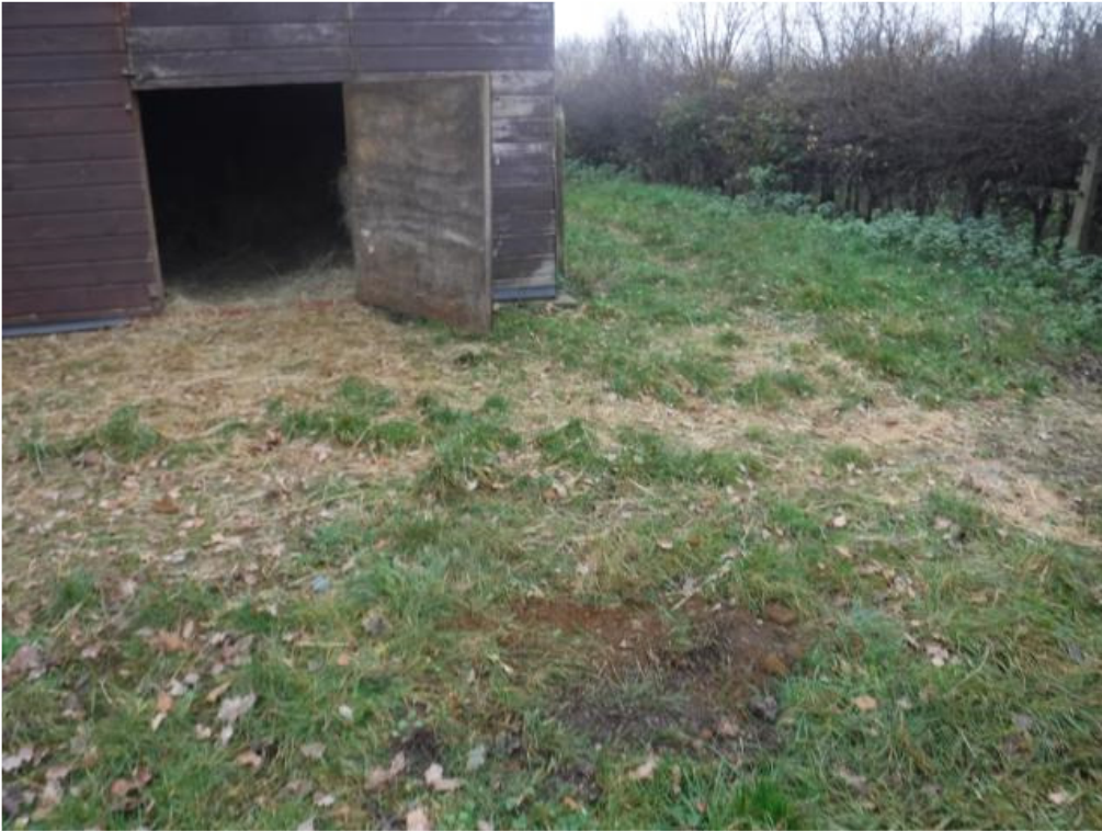
HP2 location, North of the Stable Block.
