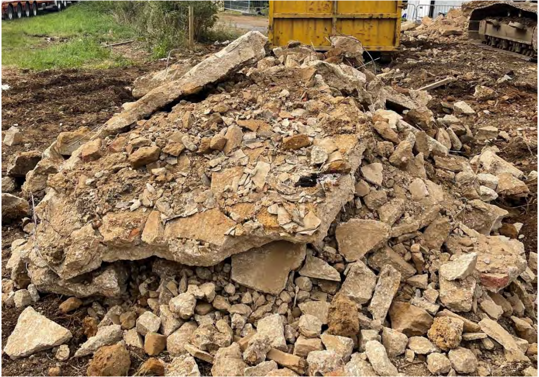
Plate 1: Asbestos cement sheets on underside of barn floor slab.
