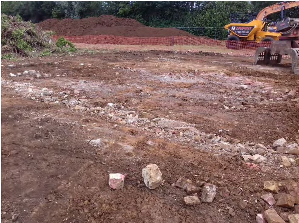
Plate 4: Exposed reworked quarry soils beneath hardcore. Flush with surrounding levels.
