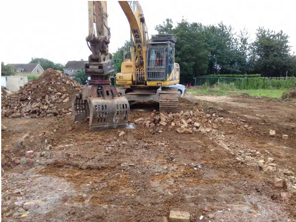
Plate 3: Scraping up of underlying hardcore layer beneath barn and track.
