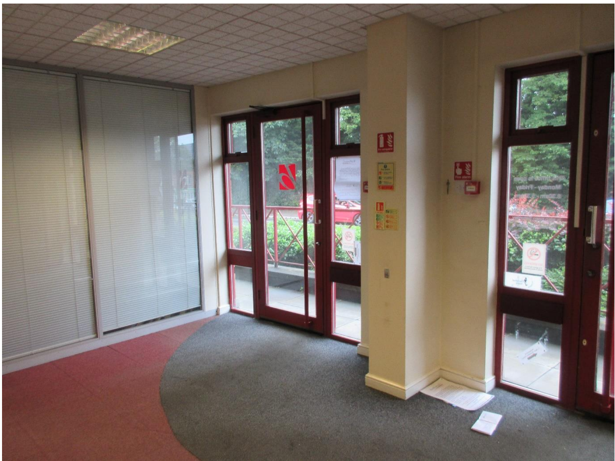
Office entrance foyer
