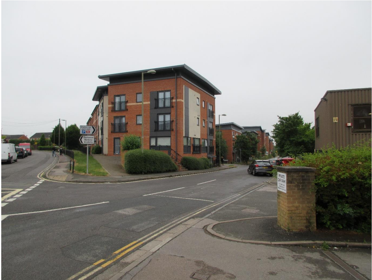
New apartment blocks opposite the entrance to the car park of the subject property
