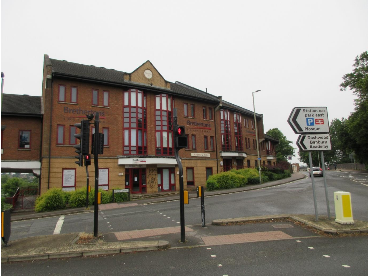
Front Elevation of Waterperry Court
