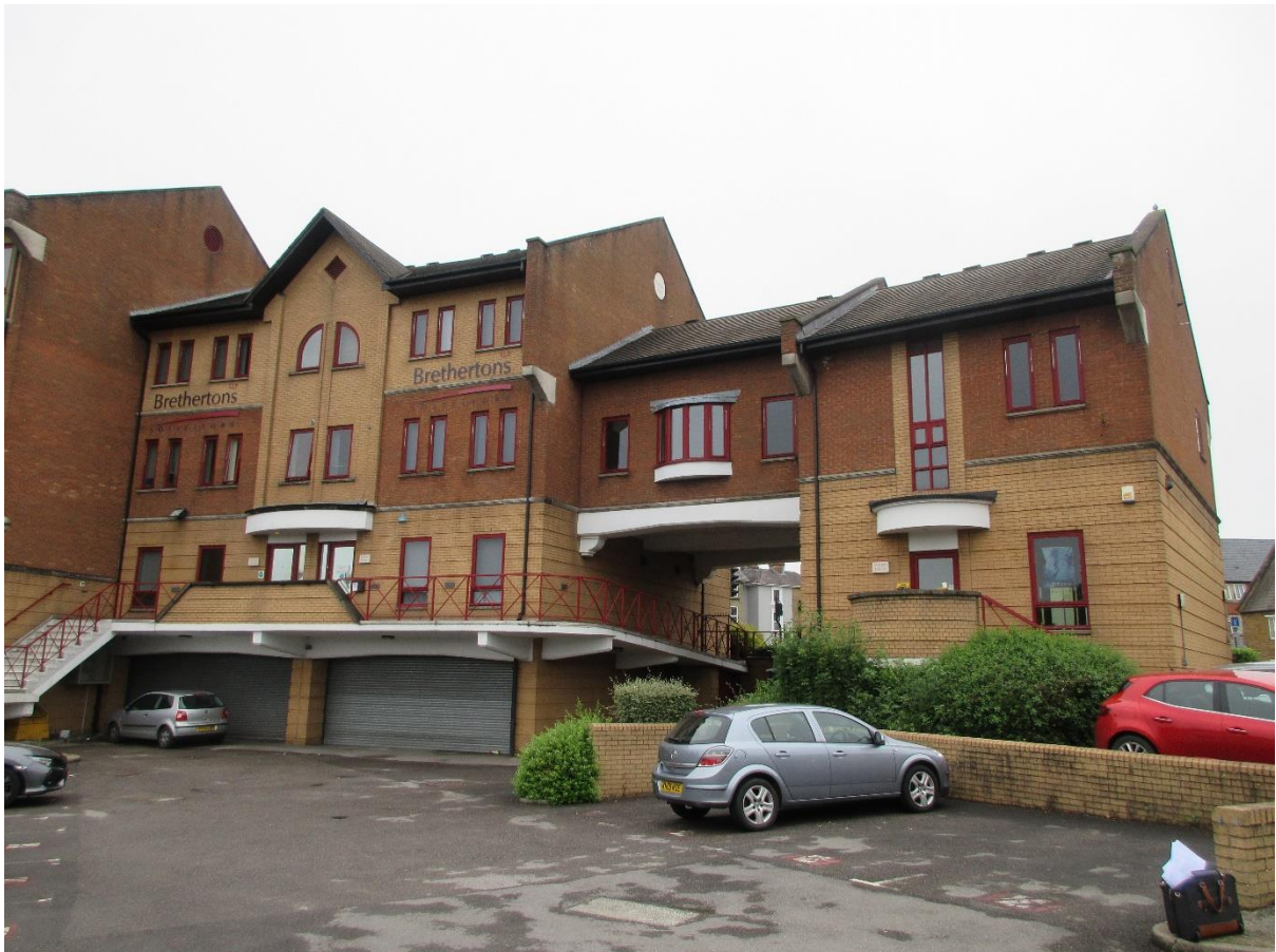
Rear Elevation showing Malvern, Buxton & Chiltern Houses
