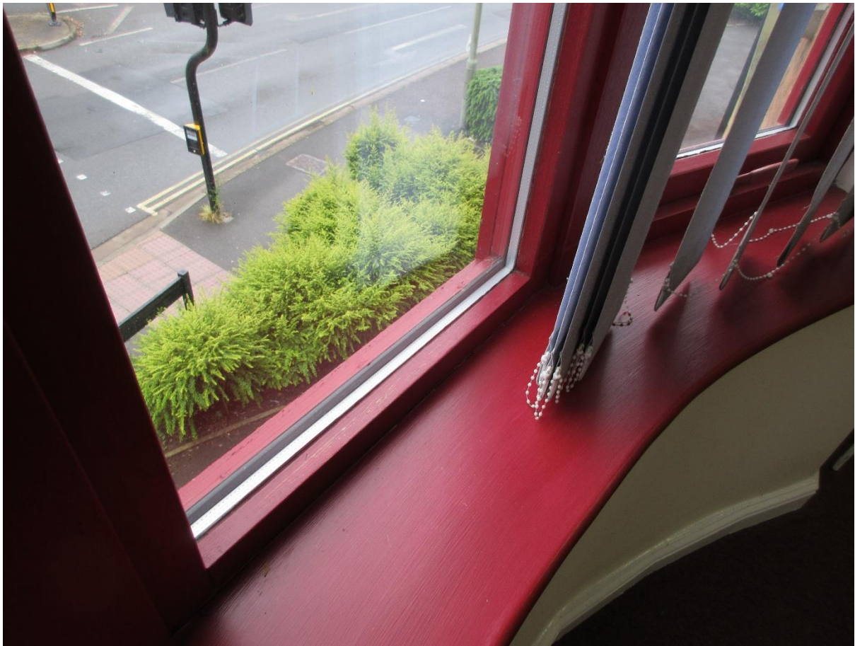
Painted timber double-glazed windows
