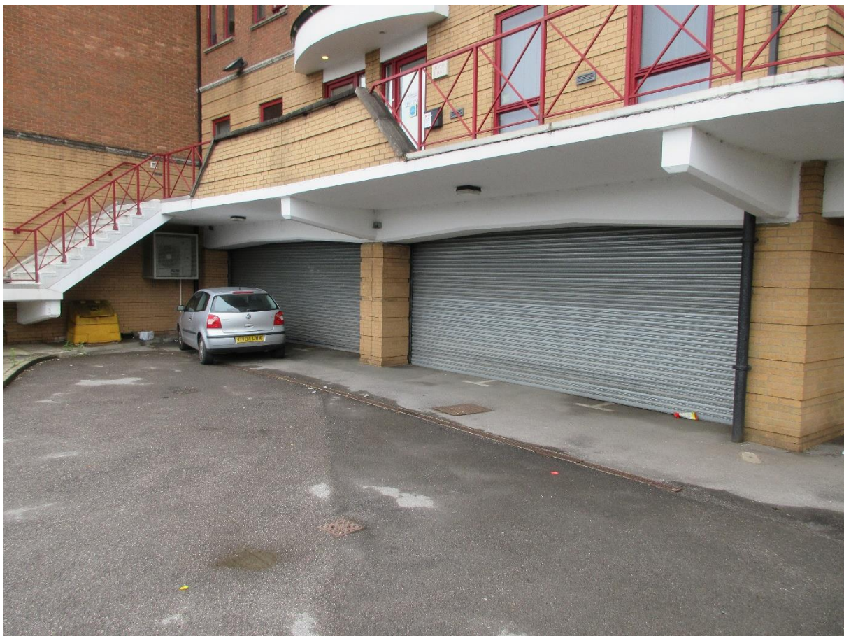
Basement parking / Storage
