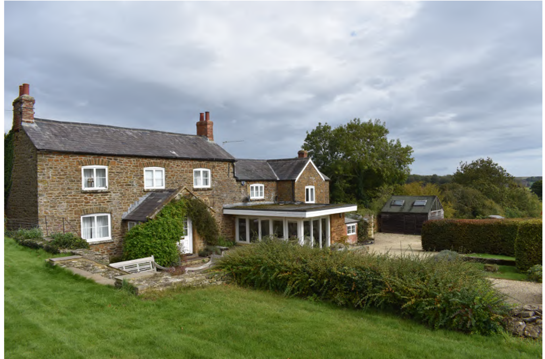
Fig. 2 - Photo of the existing property with its blue grey slate roof
