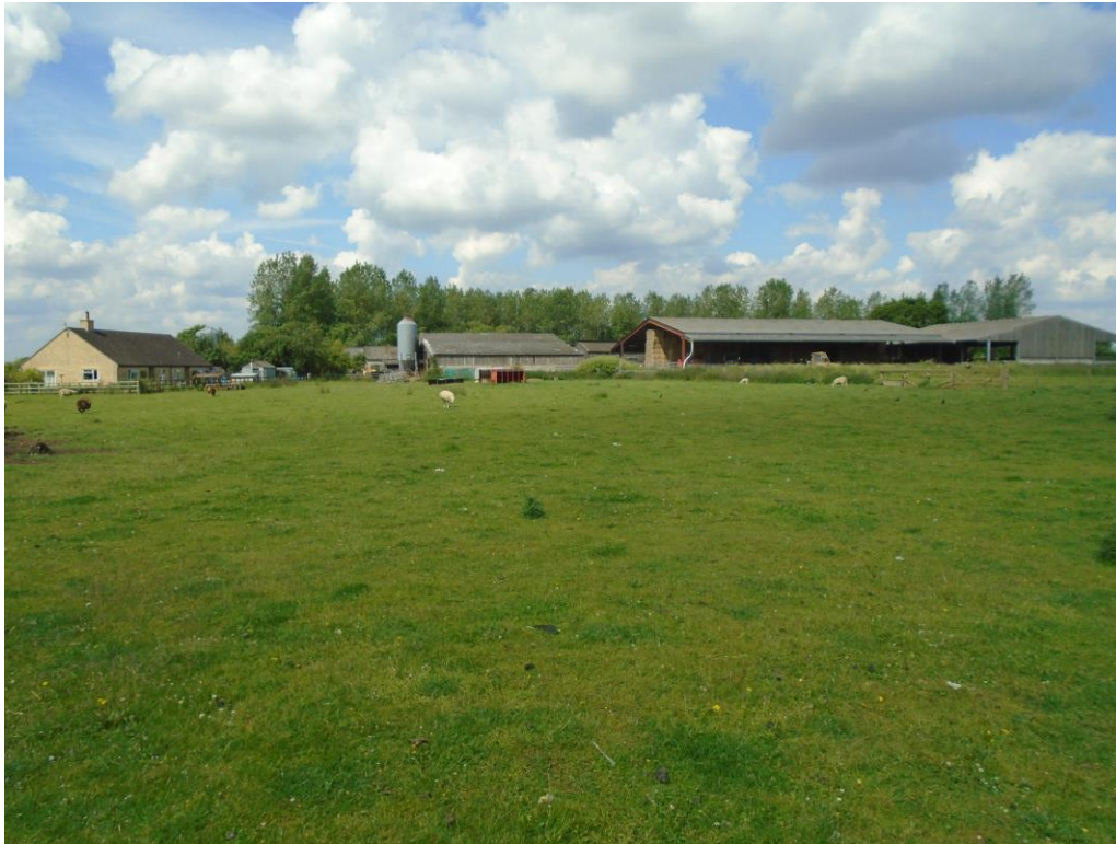
Central part of application site, looking west
