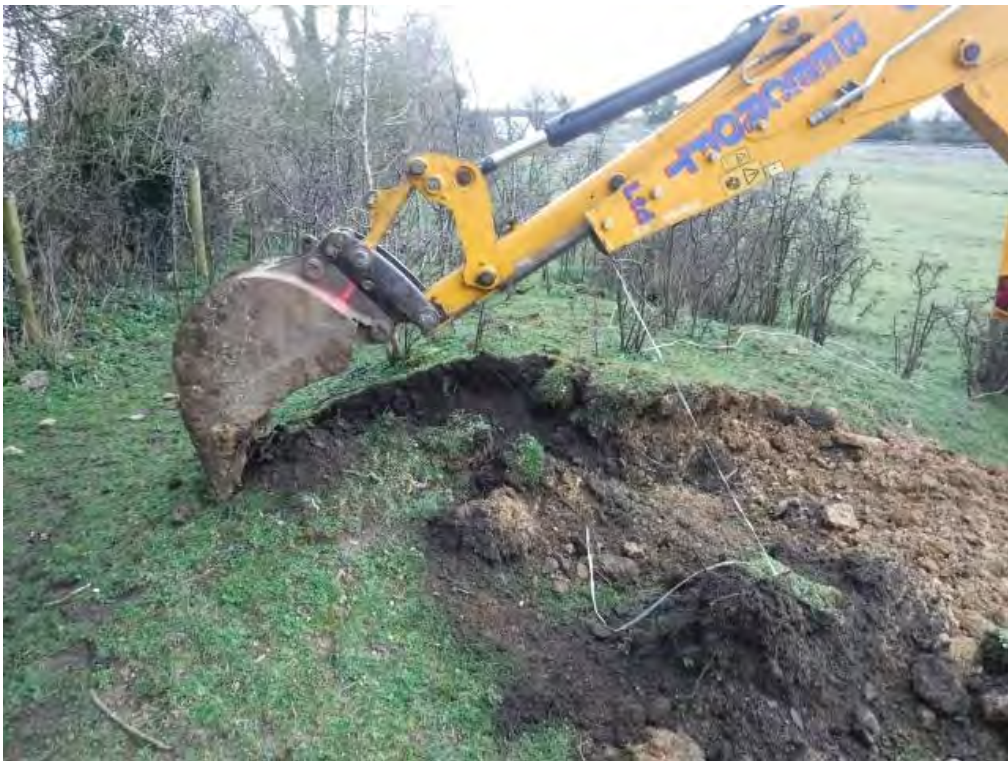
TP27 – Stockpile in North-West Corner
