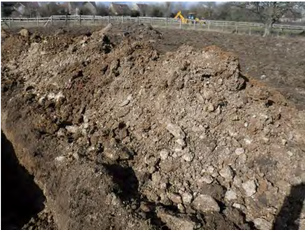
Trial Trench TP15 stockpiled arisings
