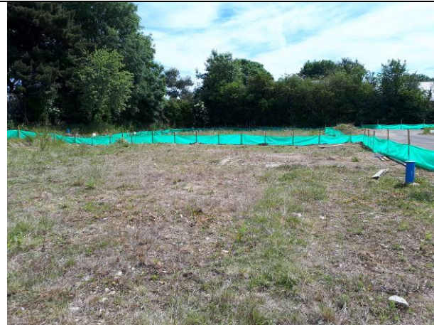
02.06.20 – Eastern view across the northern part of the site
