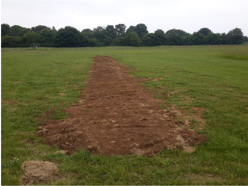
Plate 5 Backfilled Trial Pit
