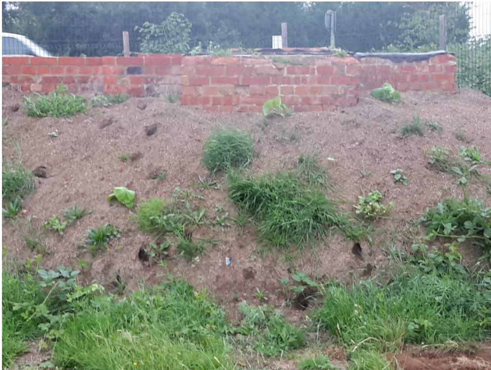
Plate 2 Former Bunker (external view)
