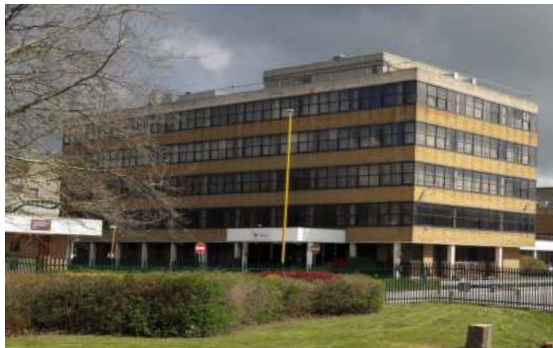
01: Demolition of the existing Main Office Block
