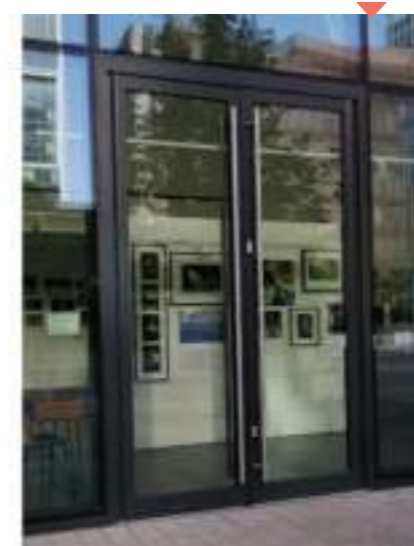
03: New double sliding entrance door
