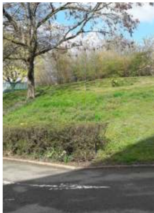
Existing embankment adjacent to car park
