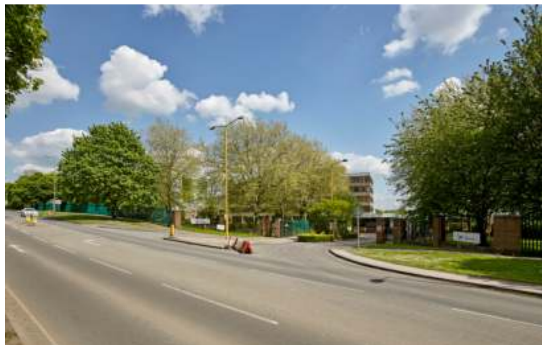
02: Existing Main Entrance View
