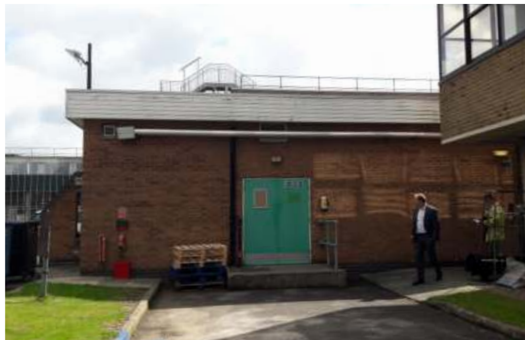
02: Recladding of Computer Suite facade
