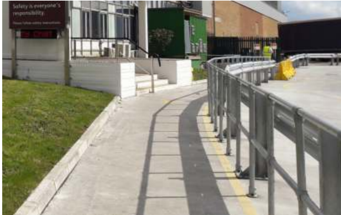
Armco barriers to separate traffic
