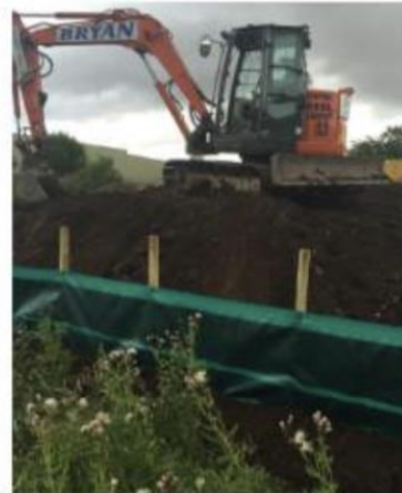
Silt Fence can be used as a temporary measure to prevent muddy water escaping from construction sites
