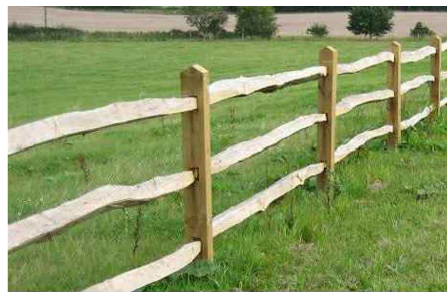
TYPICAL MORTICED TIMBER POST AND RAIL FENCE
