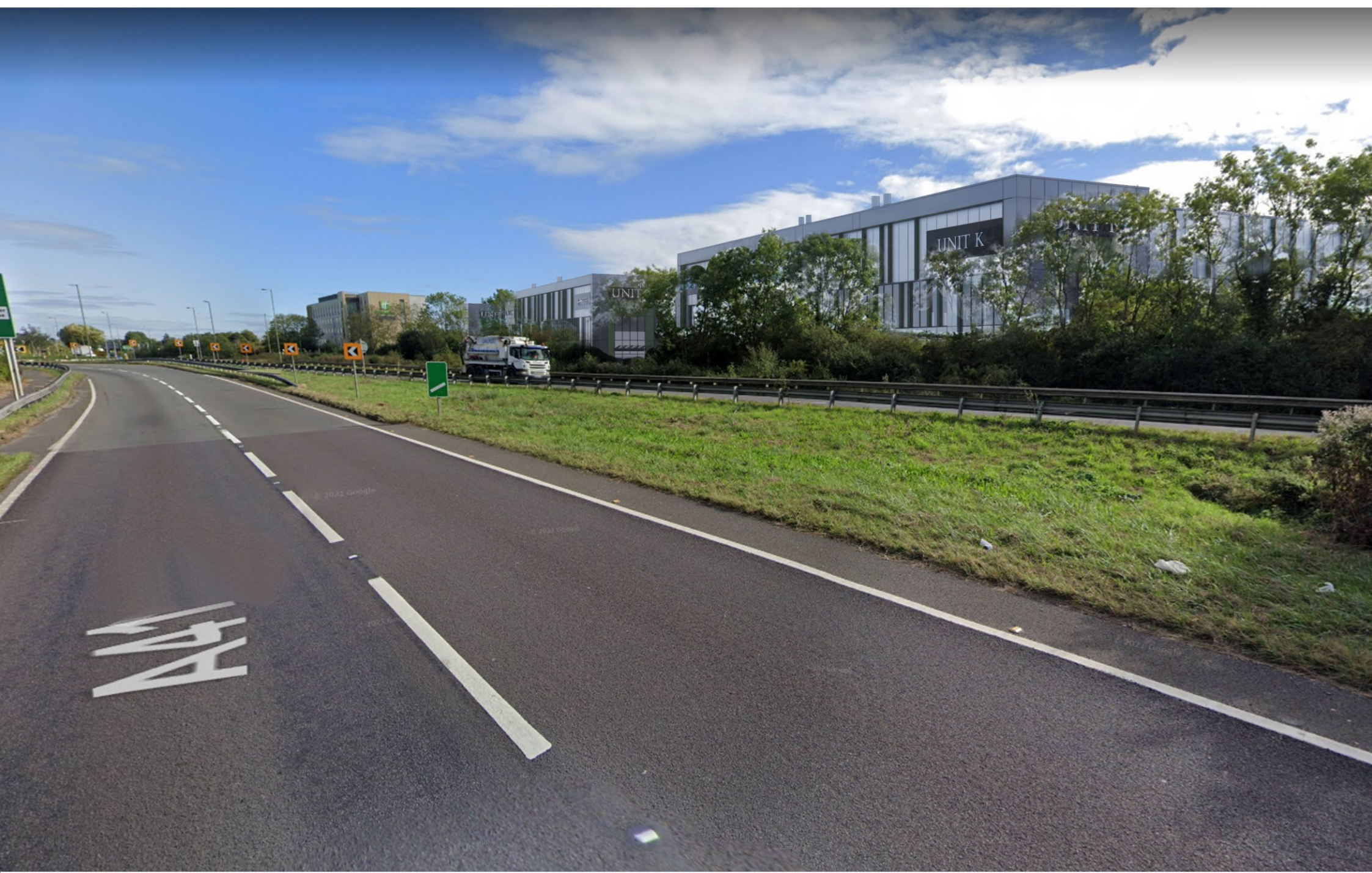
View from south approaching Unit F
