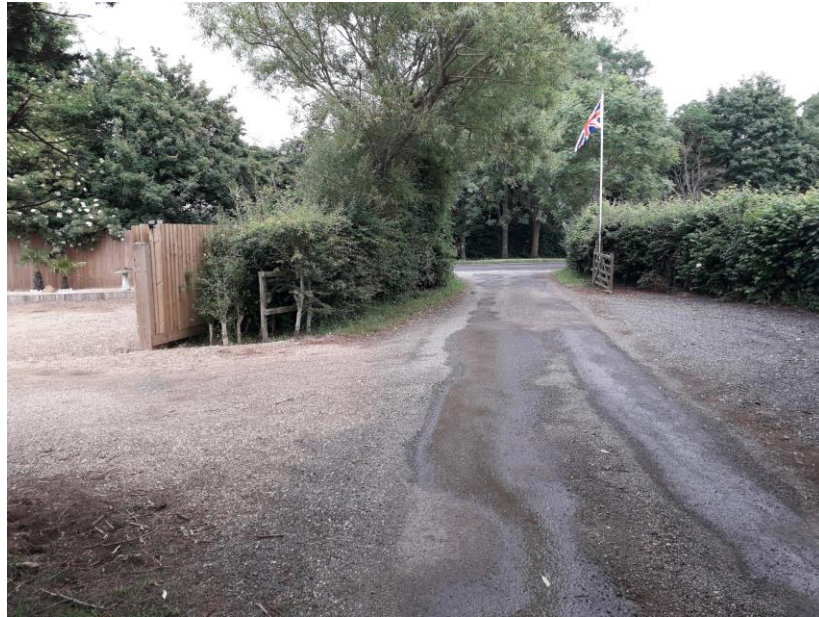
Existing access from road and into site car park
