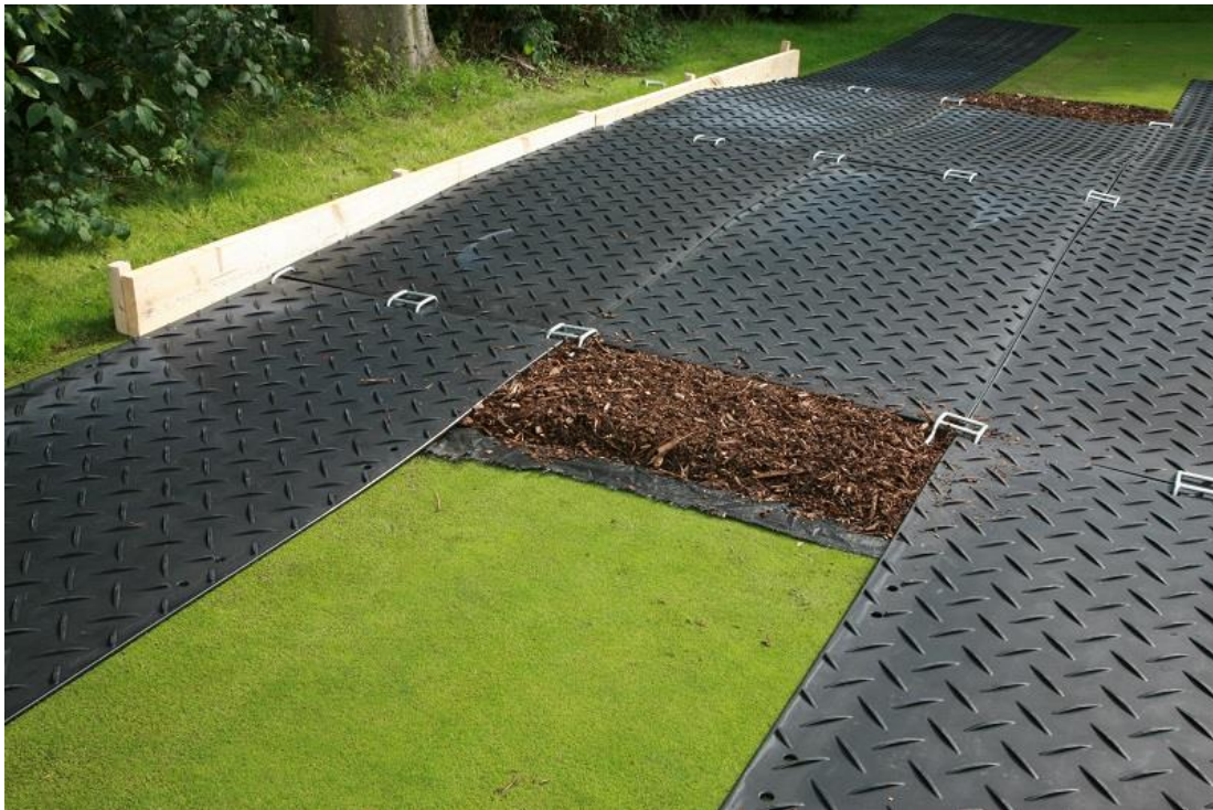
Fig. 2 Ground protection measures
