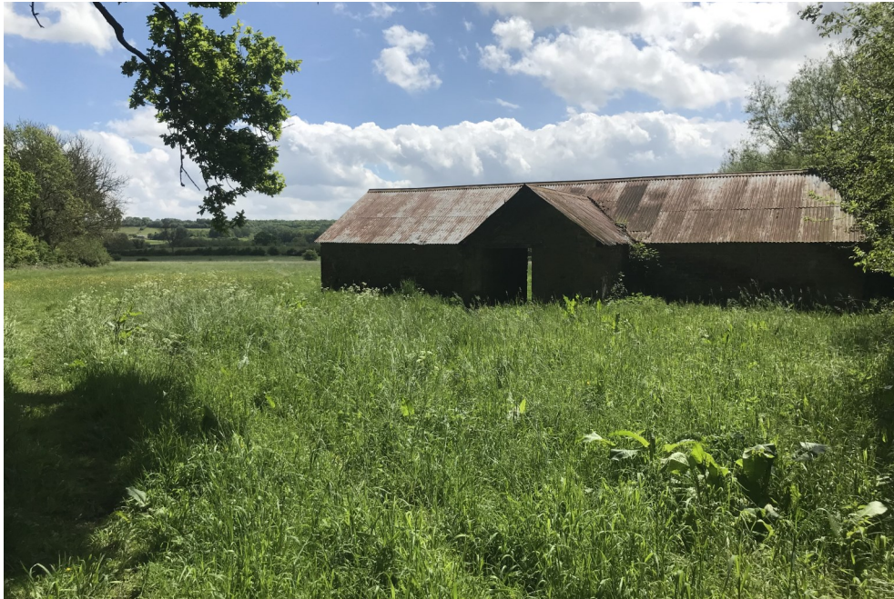
View of derelict barn on southern area of site (Area 2)
