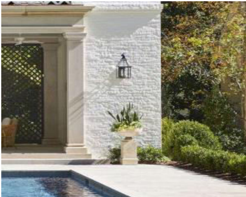
Walls – Lime wash walls.
